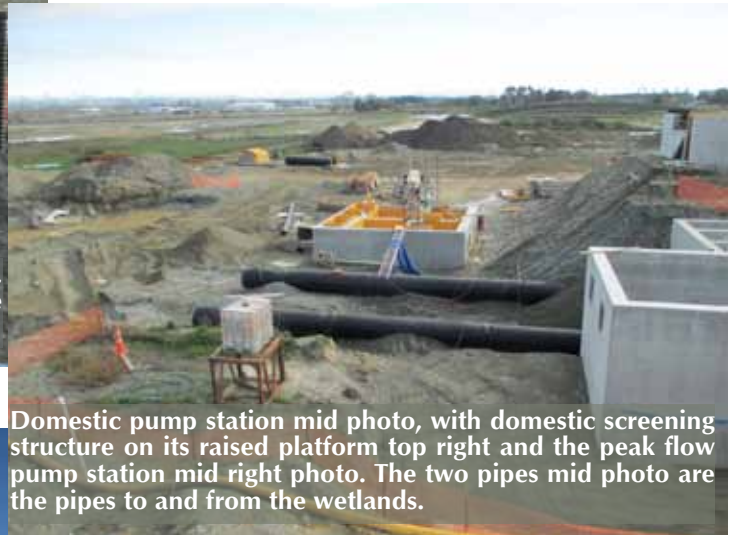
The domestic screening structure on its raised platform, with the peak flow pump station structure in the foreground
