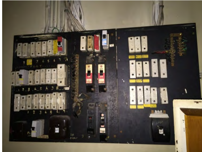
Photo 1 Typical Existing Switchboard
