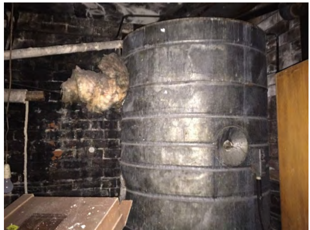
Photo 2 Original Heating Water Cylinder
