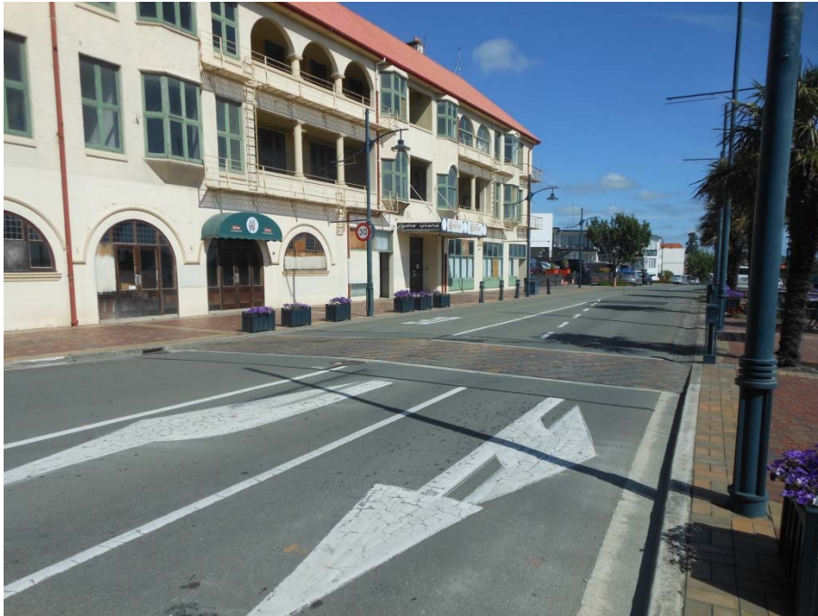
Photograph 4: Ramp and Raised Platform on The Bay Hill
