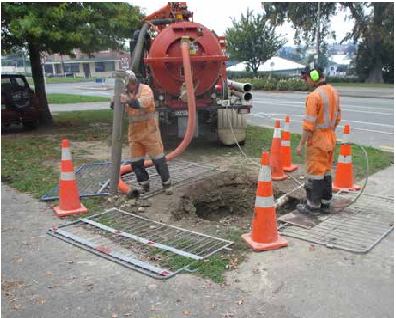
Church Street Sewermain Renewal
