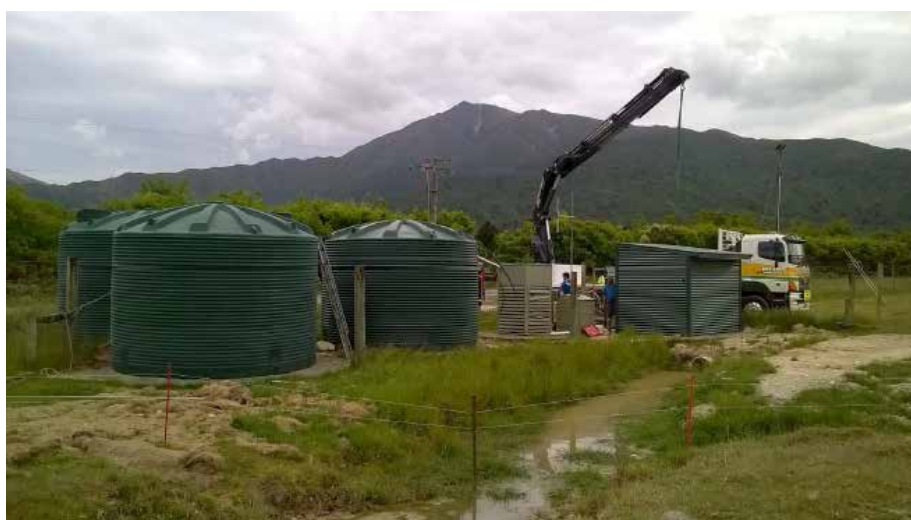
Peel Forest Water Storage
