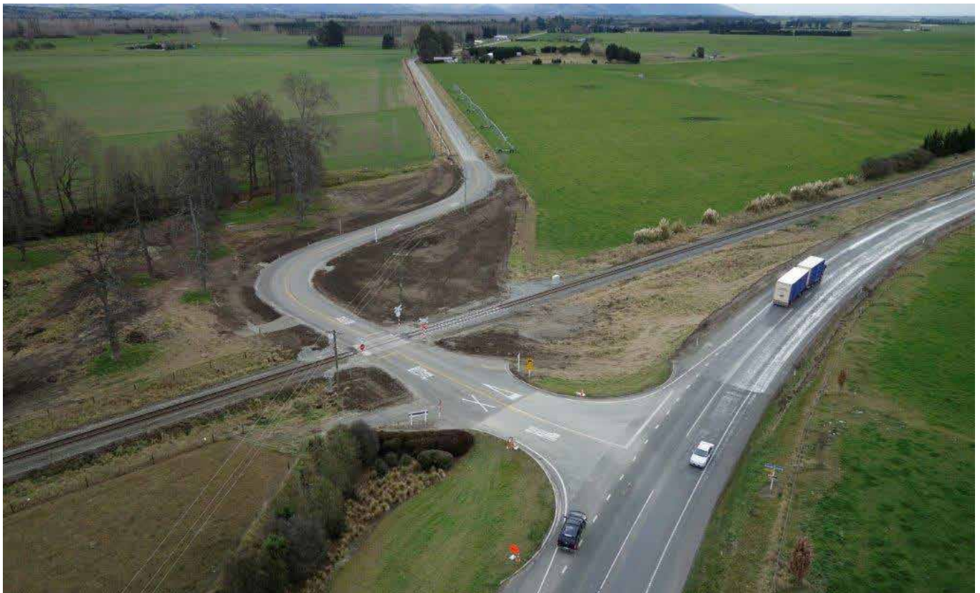
Arundel Belfield Road Realignment
