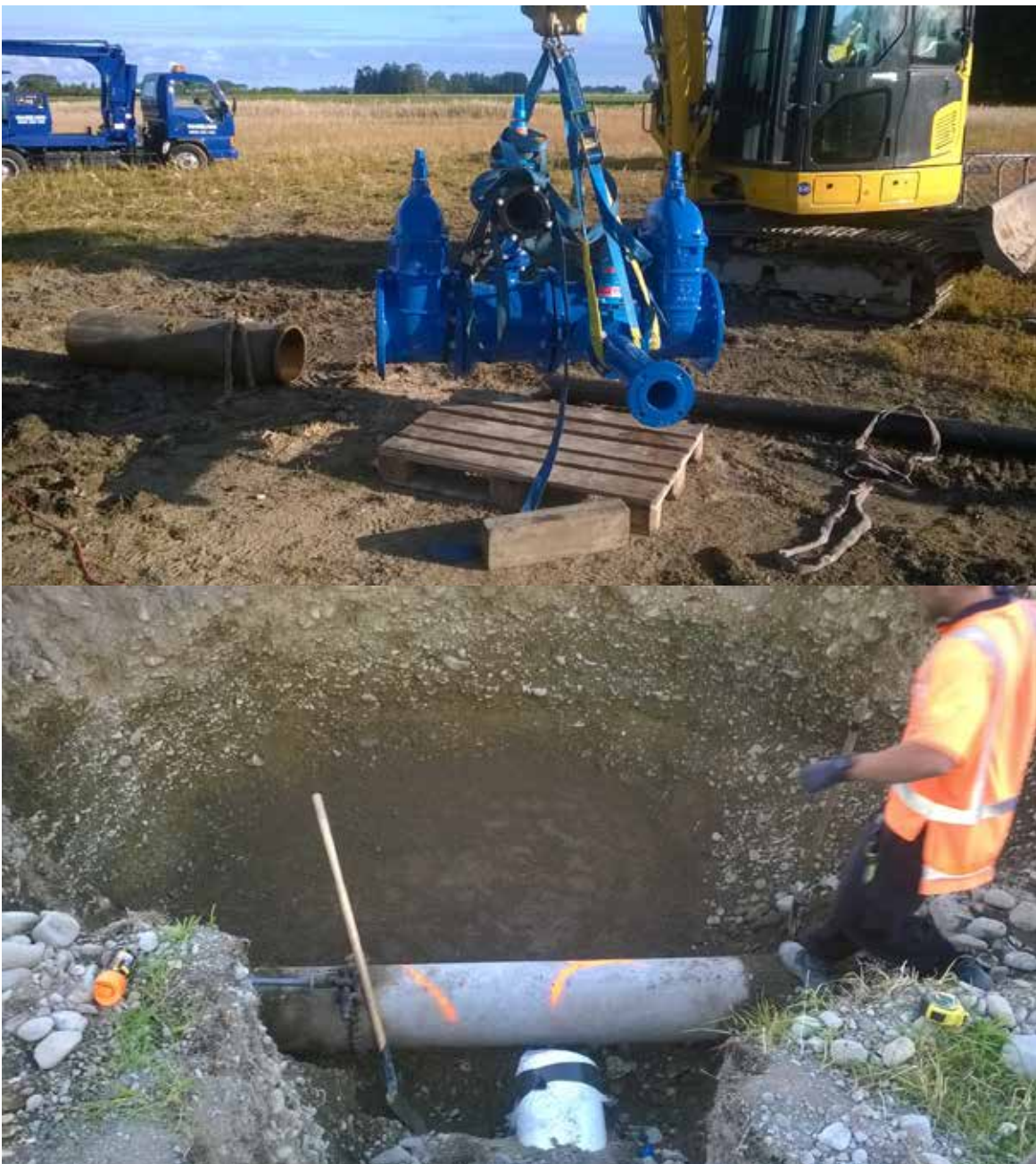
Replacement of 3.8km of trunk water main December 2015
