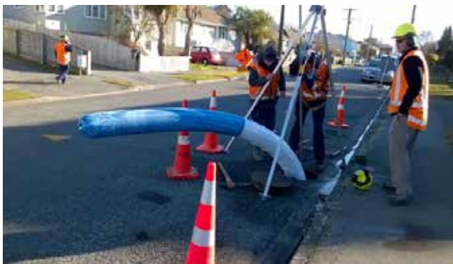
Canada Street Sewermain Rehabilitation
