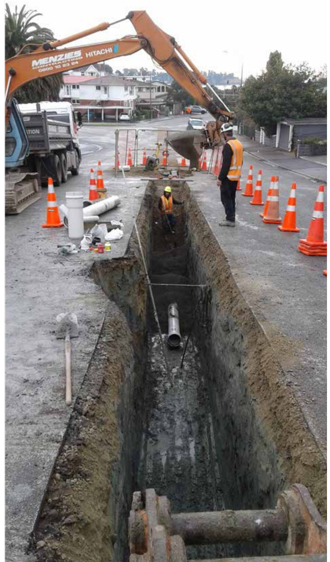
Hewling Street Sewermain Renewal
