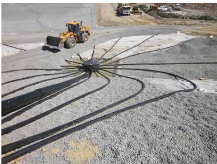
Redruth Landfill Cell 3.4 Construction - Leachate System
