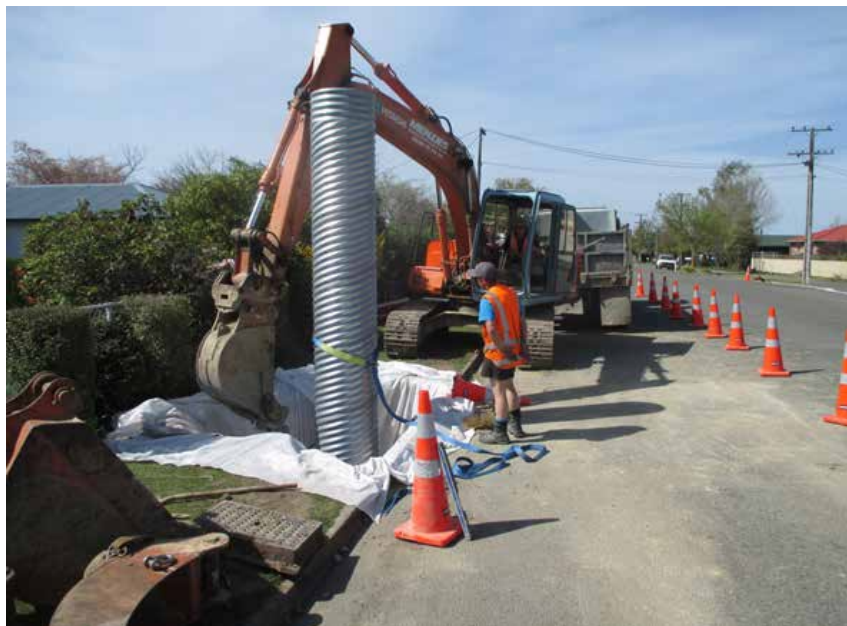
Connolly Street Soakpits Renewal
