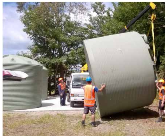
Winchester Water Storage
