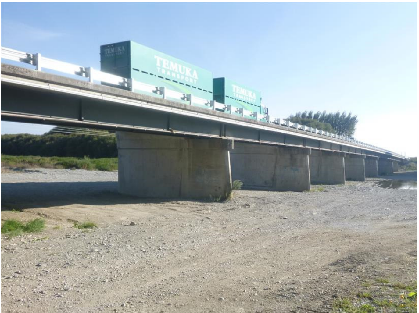
Badhams Bridge Widening
