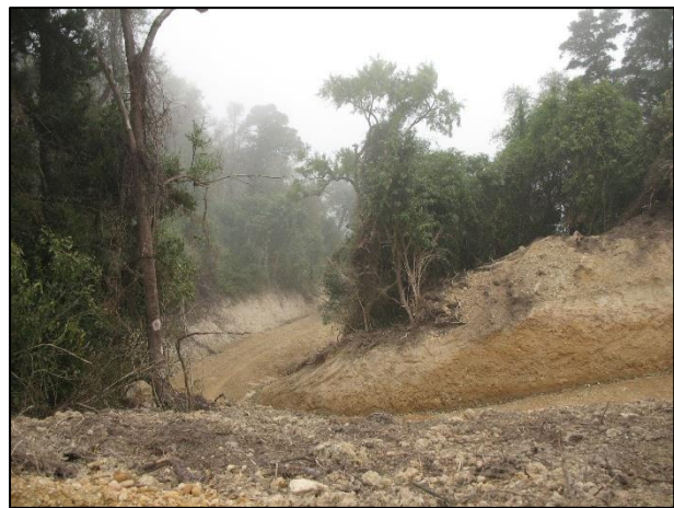
Vegetation clearance on Geraldine Downs
