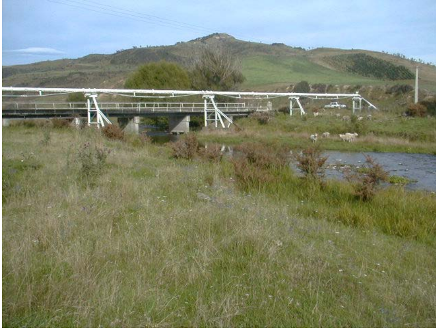
Pareora Pipeline - Pipe Bridge
