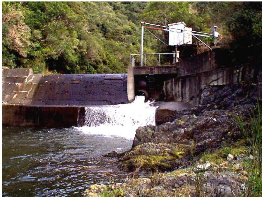
Intake weir with scour valve open
