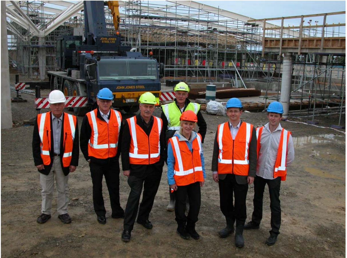
The Timaru District's Mayor and some councillors enjoyed a close-up view of the new Caroline Bay Aquatic Centre this week when taken on a tour of the construction site by district services manager Ashley Harper and Ranger Construction Ltd construction manager Simon Harding. Pictured in front of the rapidly-developing centre are (from left) Cr Richard Lyon, deputy mayor Cr Michael Oliver, Cr Pat Mulvey, Mayor Janie Annear, Ranger Construction manager Simon Harding (at rear), Cr Steve Earnshaw, and Cr Hamish Fraser.
