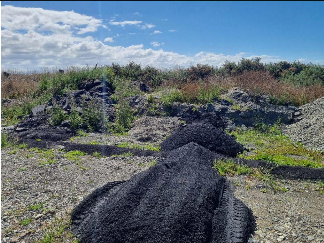
Photograph 19: Hardfill and road millings and asphalt surplus stockpiled in the east of the Seadown firing range complex for use on site for roading (5-Mar-2025).
