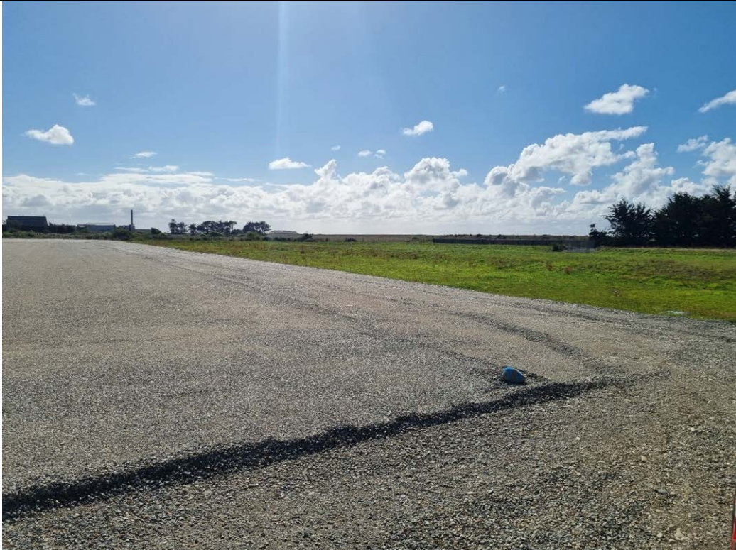
Photograph 7: View east from the new building pad towards stormwater ponds in rear of Hilton Haulage yard at 144 Meadows Road (5-Mar-2025).
