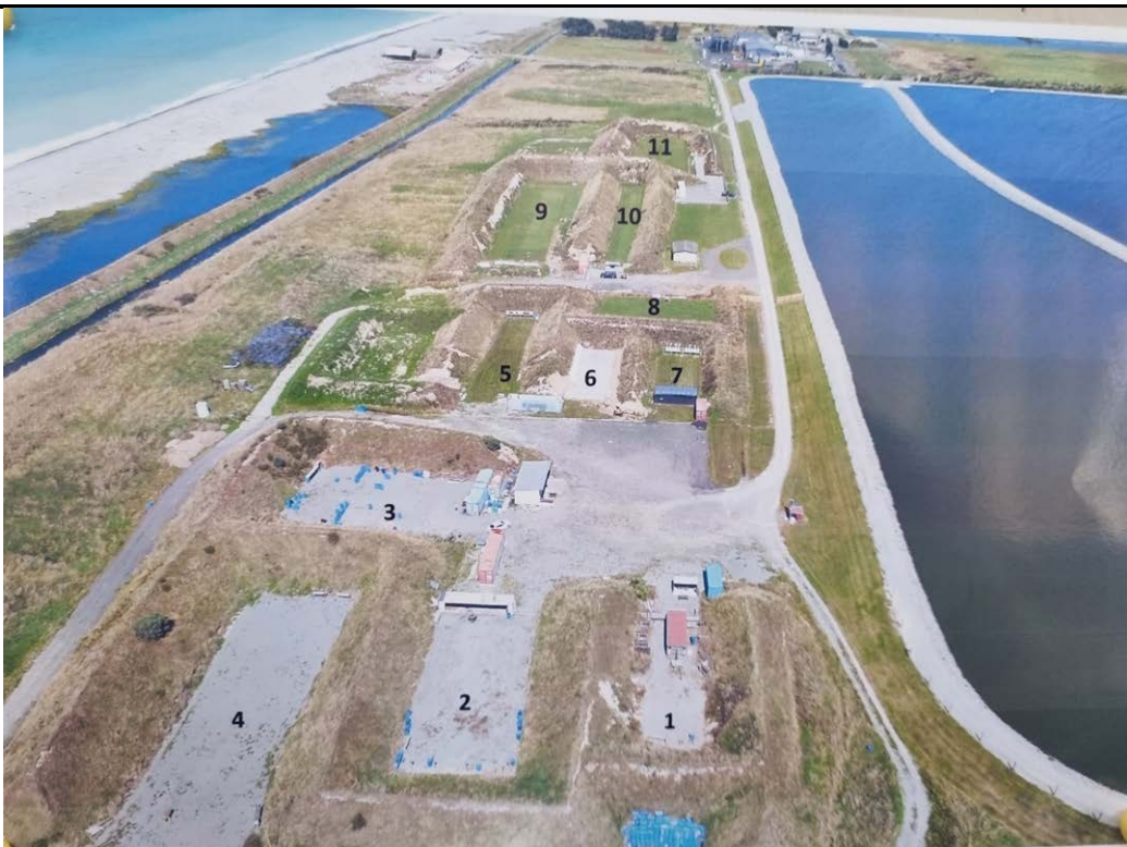
Photograph 16: An undated aerial photograph of the Seadown range complex, view southwest with gun range identification numbers presented (16-Apr-2025).
