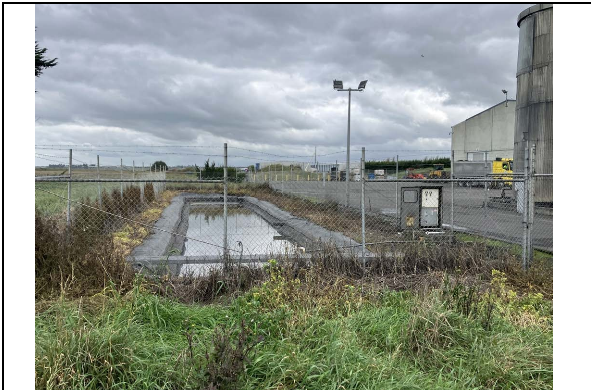
Photograph 29: Wastewater pond 124 Aorangi Road (Lot 2 DP 419868) (16-Apr-2025).
