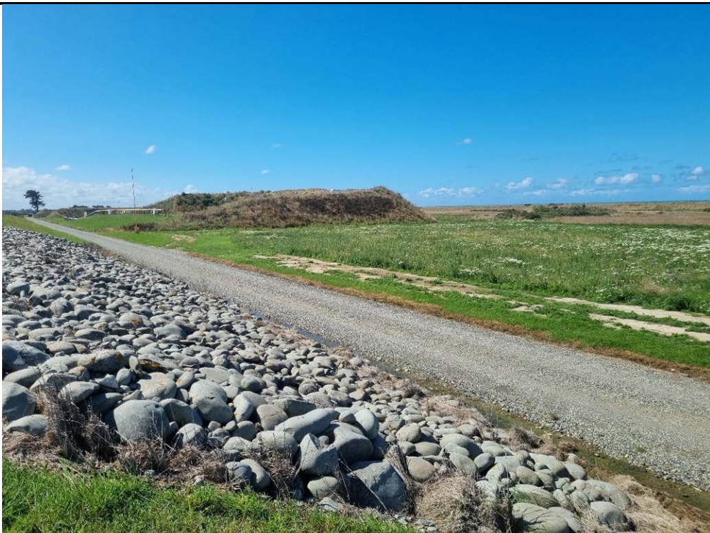
Photograph 24: View north from western boundary of TDC land leased to Seadown Shooting Complex. TDC wastewater pond spillway visible in foreground and to left of photograph (5-Mar-2025).
