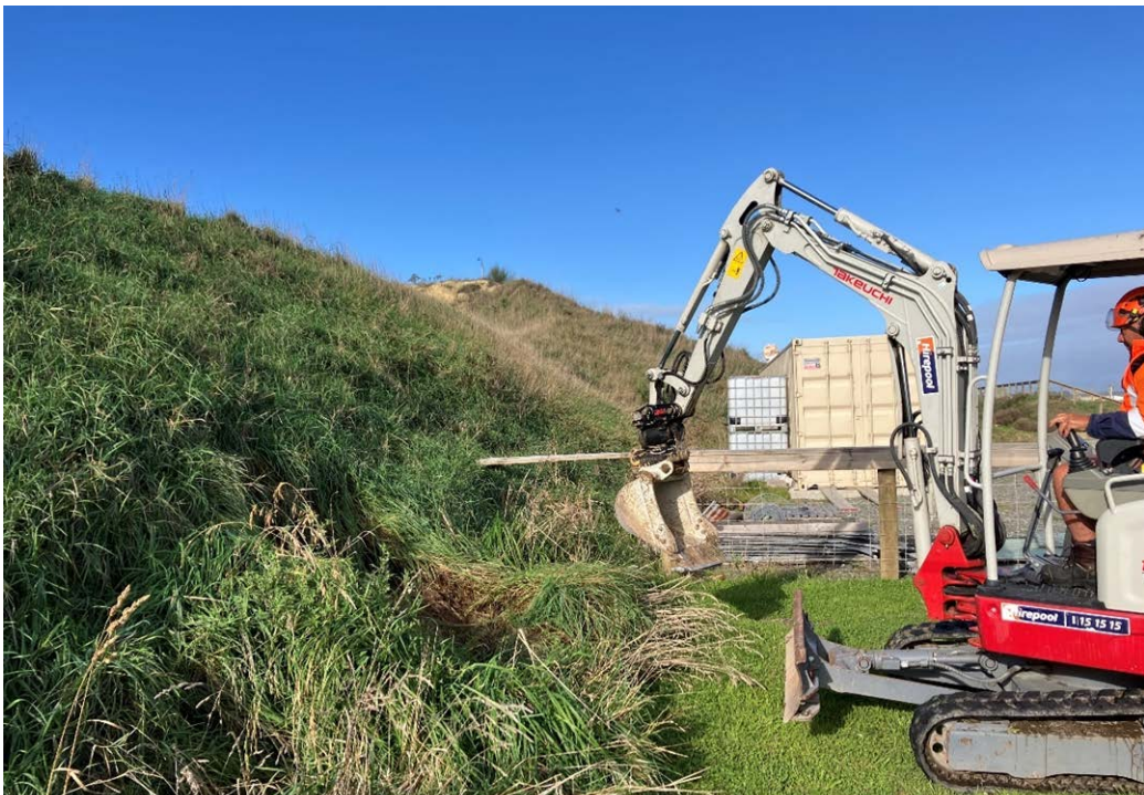
Photograph 20: Example of bunding at Gun Club (16-Apr-2025).
