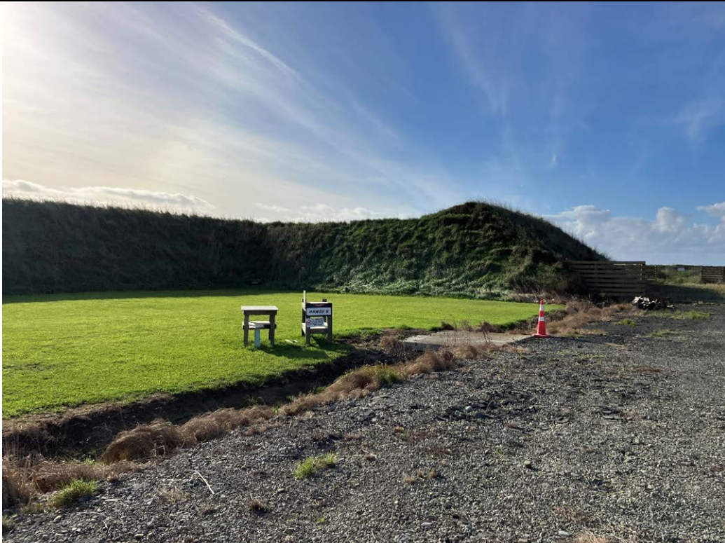
Photograph 21: Example of bunding at Gun Club (16-Apr-2025).
