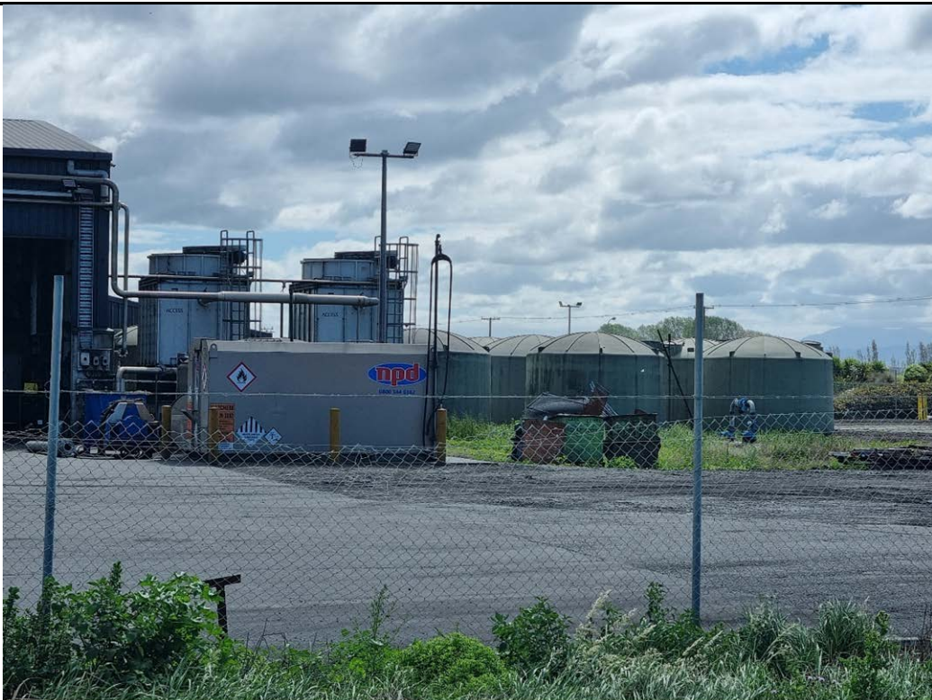
Photograph 32: View northwest of an above ground diesel storage tank on the By Products site (5-Mar-2025).
