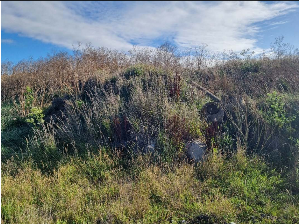
Photograph 5: Stockpiles in southern half of 72 Sheffield Street containing concrete and treated timber poles (5-Mar-2025).
