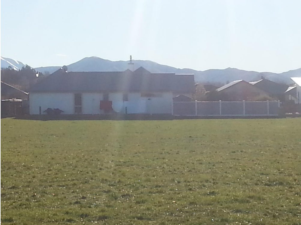
Horrell Residence, 15 Cascade Place (Support)
