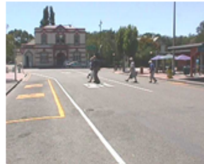
Junction 3 no pedestrian crossing facilities
