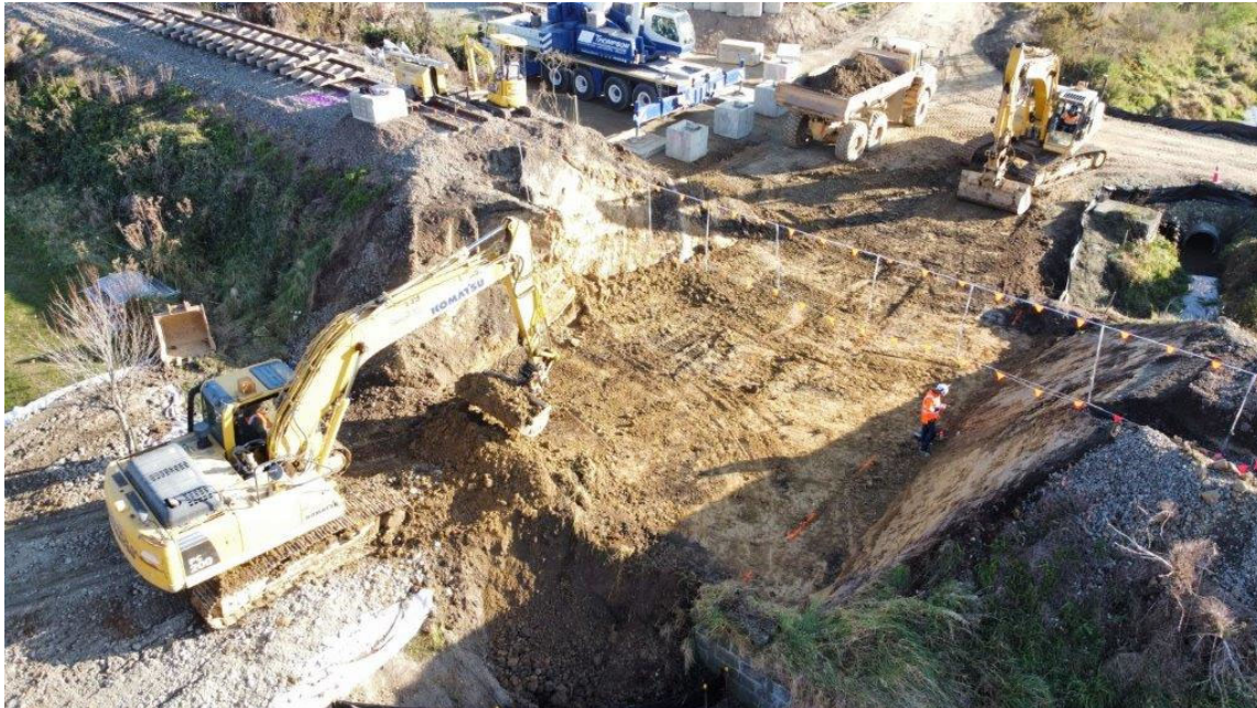
Taitarakahi Creek new culverts under construction.
