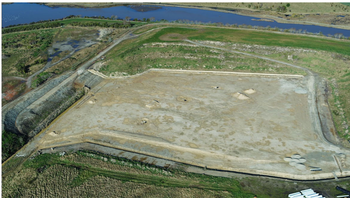
Redruth Landfill Cell 3.5 Under Construction – Photo taken 12 August 2022
