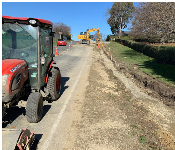
Washdyke Water Network Improvement Stage 1.
