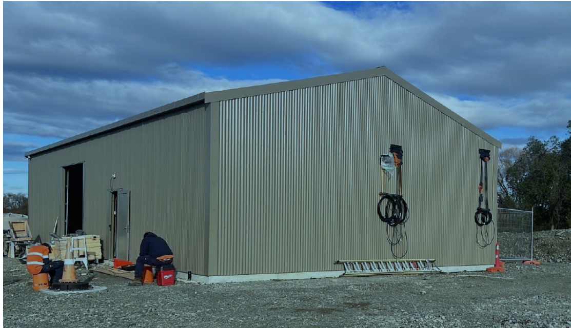
Exterior of Te Moana Water Treatment Plant
