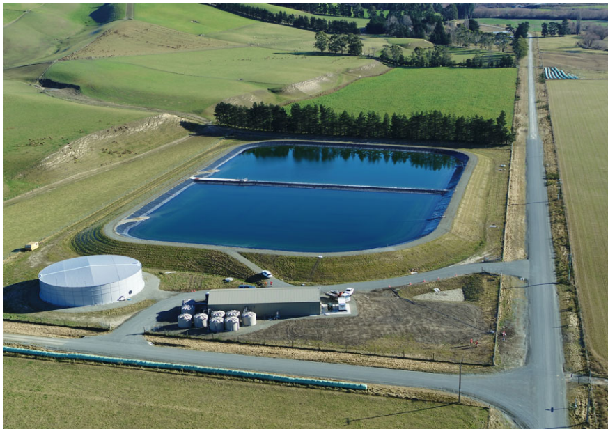
Drone photo of Te Ana Wai Water Treatment Plant, Treated Water Reservoir and Raw Water Storage Ponds.
