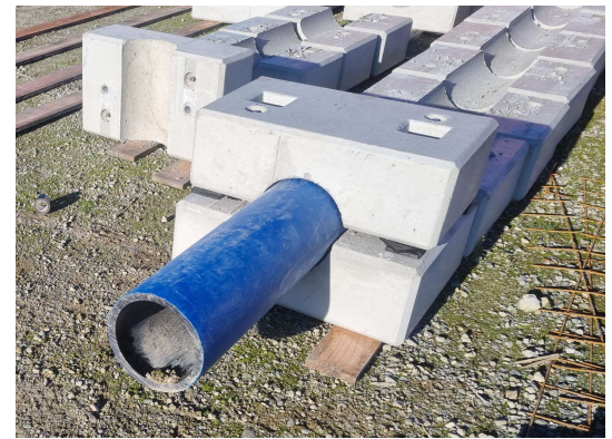
Left: Installing Bat detectors. Middle: Juvenile Lamprey found on site. Right: Ensuring Anti-Flotation Blocks are the right fit for the size pipe being used..
