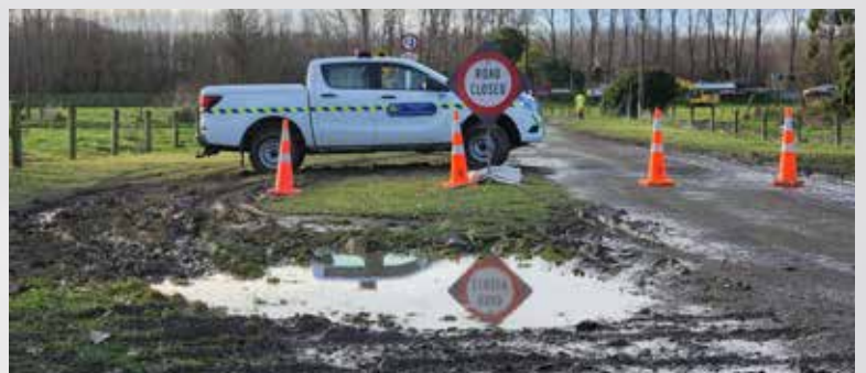
Road closure and stopbank scouring, caused by the state of emergency level flooding of the Opihi River resulting in the evacuation of the Mill Rd settlement
