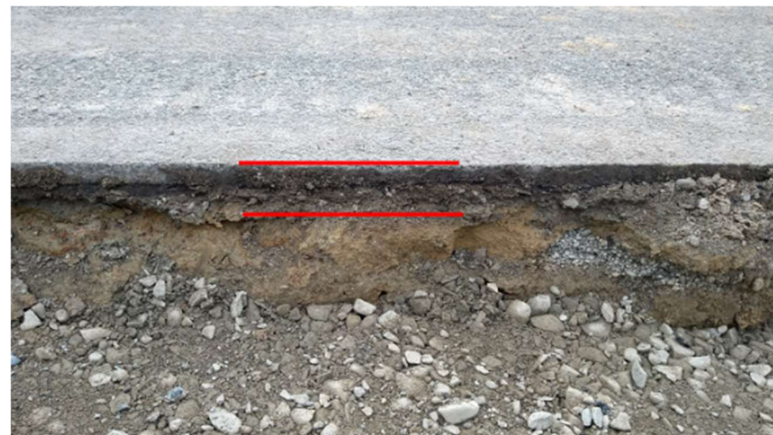
Fig. 50: Typical pavement thickness on a rehabilitation site (50-70mm)
