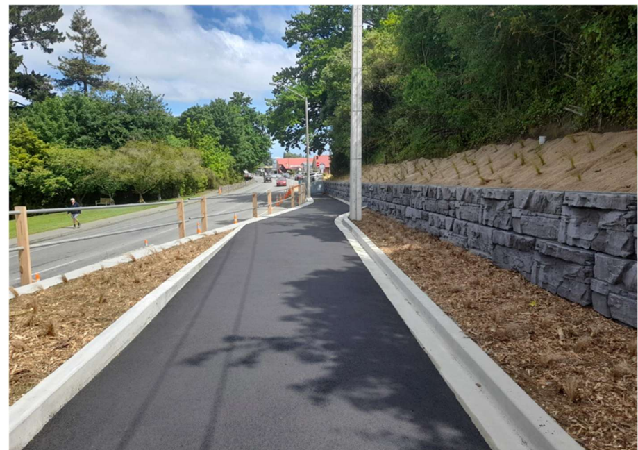
Fig 92: Coulter Place, Geraldine – a new retaining wall has been installed in 2023. This was an important resilience upgrade for State Highway 79, but funded by Council due to proximity to the footpath.
