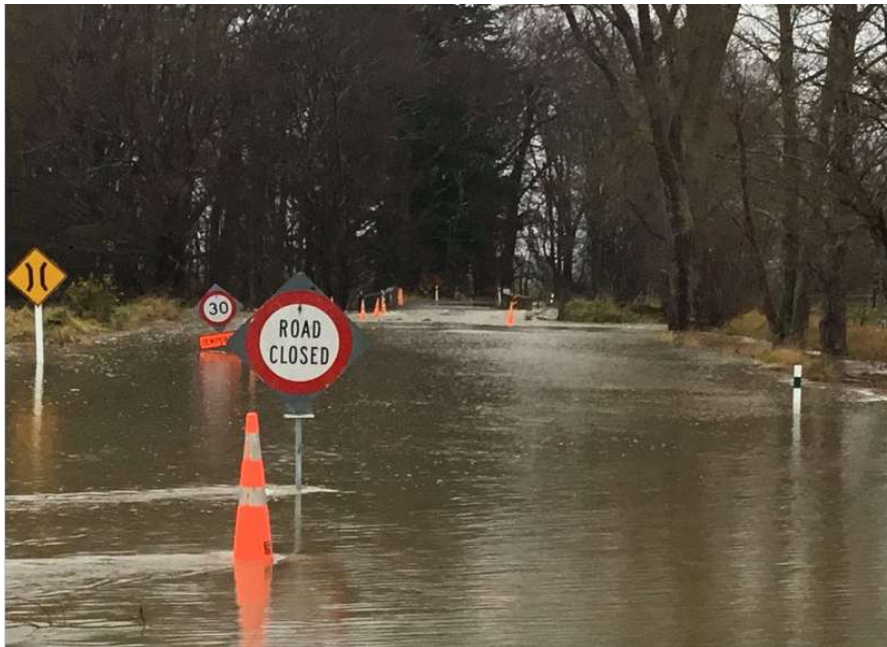
Fig. 94: Flooding at Langridge Road bridge – we have received resilience upgrade requests for this location. The existing structure is not near the end of life, if project was to be brought forward it would require full Council funding including a full assessment of flow paths.
