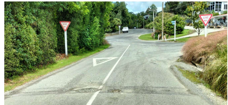
Fig. 20: Waihi Terrace, Geraldine - poor reinstatement jobs reduce the life of roading assets.
