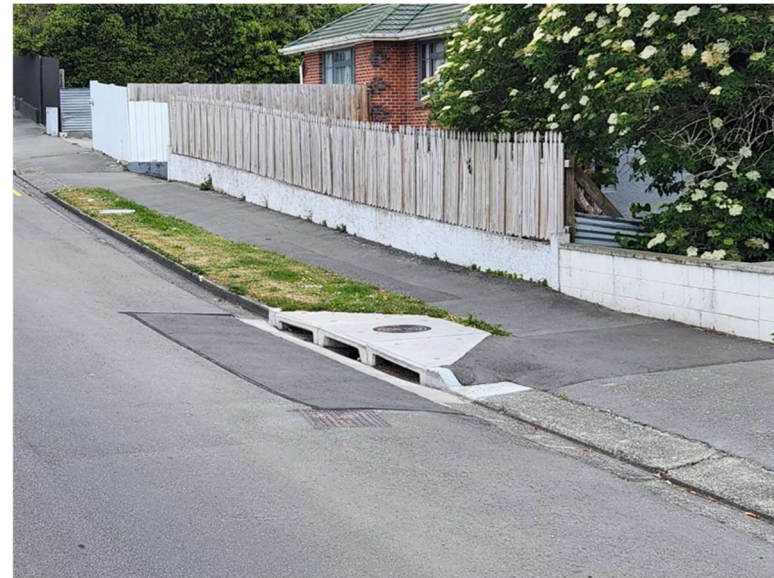
Fig. 81: A recent sump renewal in urban Timaru, to address flooding issues in this flooding depression area. This asset will rely on the capacity of stormwater mains at this location which were not renewed.
