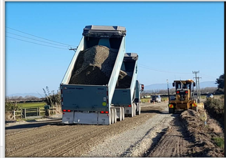
Fig. 16: Badham Road Rehabilitation Project
