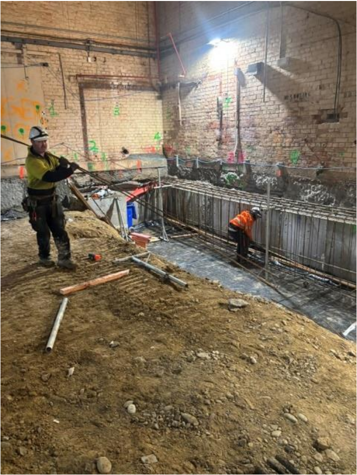
Stagehouse underpinning and foundations
