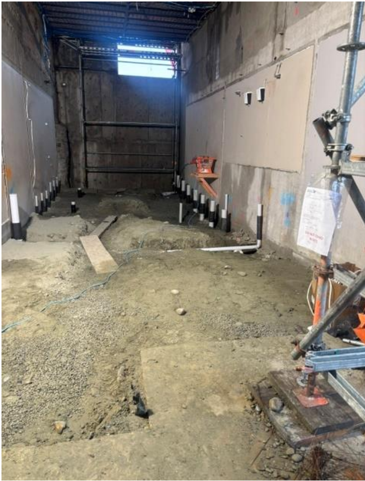
Plumbing for restrooms
