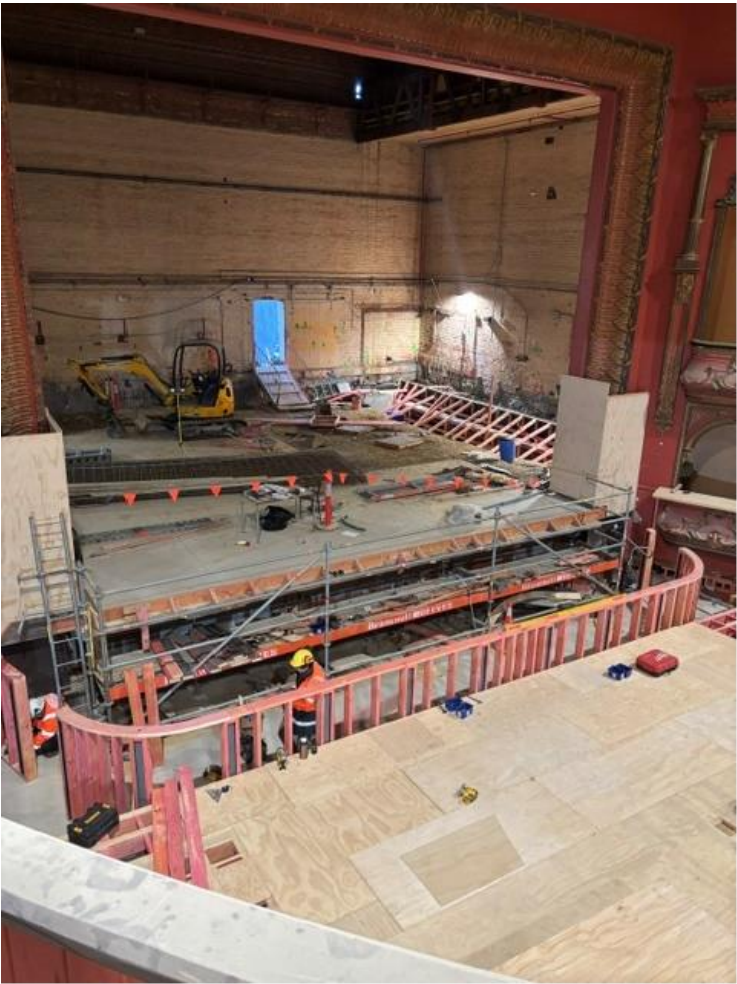
Auditorium floor and stage construction
