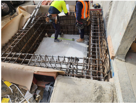
20260811_120634 – FOH lift pit.
