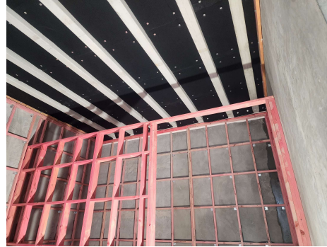
20260818_114938 - Museum Storeroom framing
