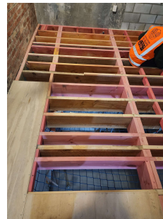
20260811_112859 - FOH first floor remediation
