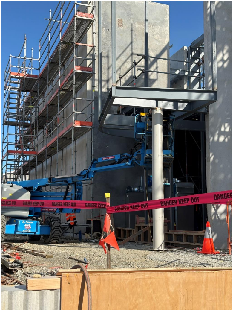
CLT Stair Supporting Steel
