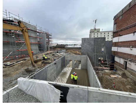
IMG_2009 – BOH Slab Prep
