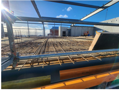
20260804_101251 - Museum Upper slab mesh
