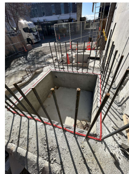
IMG_2095 - FOH Lift pit
