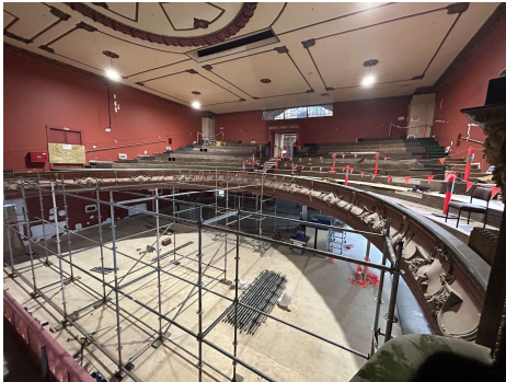
IMG_2023 - Auditorium scaffold
