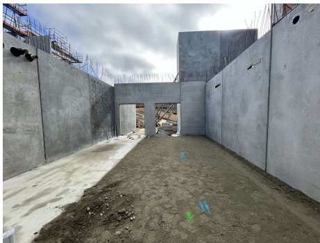
IMG_2061 – Plant Room Slab Prep
