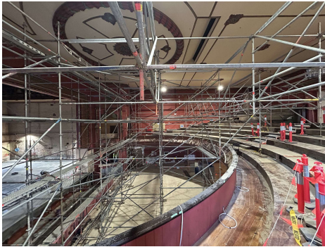
IMG_2087 - Auditorium scaffold
