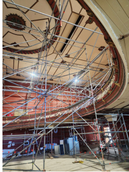
20260814_112010 - Auditorium ceiling bird cage install
