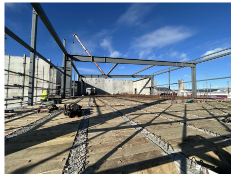
IMG_1932 – Museum Upper Floor Slab Prep
