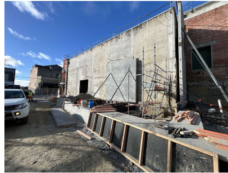
IMG_1952 – FOH Foundation beams
