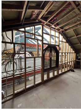
IMG_2044 – Control Room ready for fire rating
