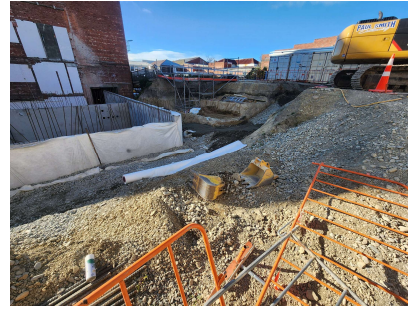
20260804_101801 - External groundworks and backfill
