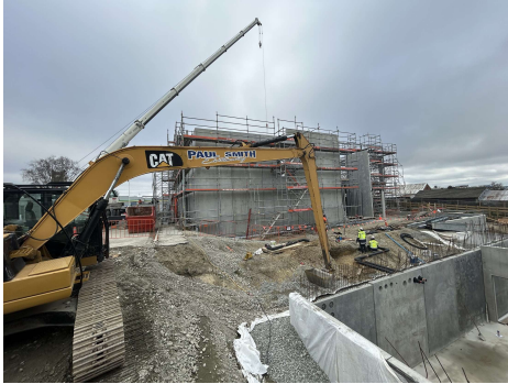
IMG_2008 – Backfilling precast
