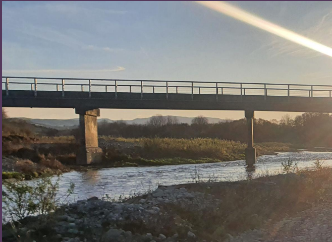
Hanging Rock Bridge
