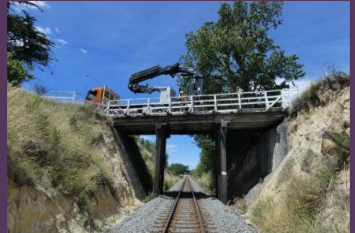
South Street Bridge - before replacement
