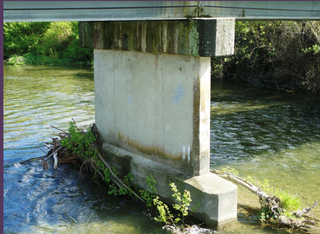
Hanging Rock Bridge - pier
