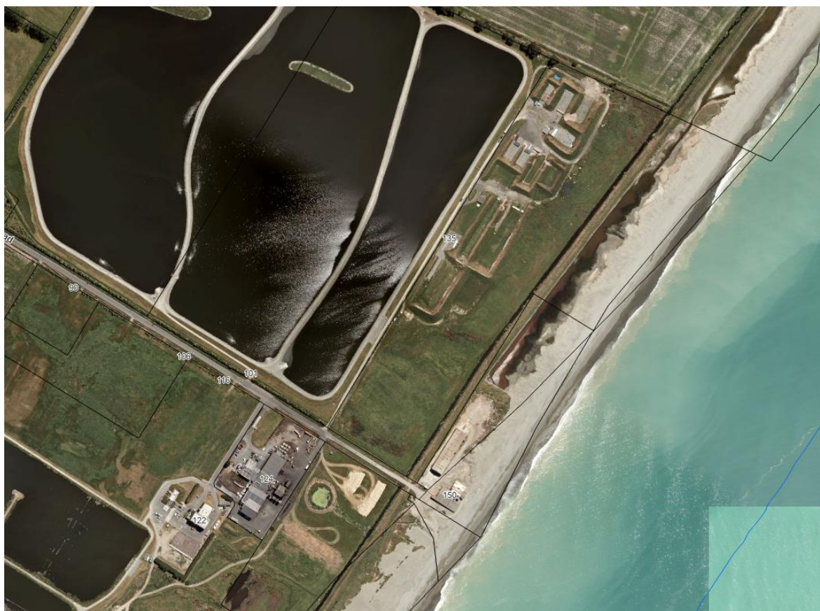
Figure 3A: Aerial photograph of existing stopbank and drain and future northern portion of Phase 1 works.
