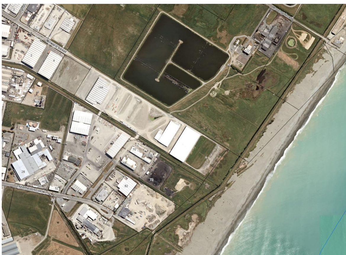
Figure 3B: Equivalent photograph of southern extent of stopbank and drain and future works (Source: Council GIS).
