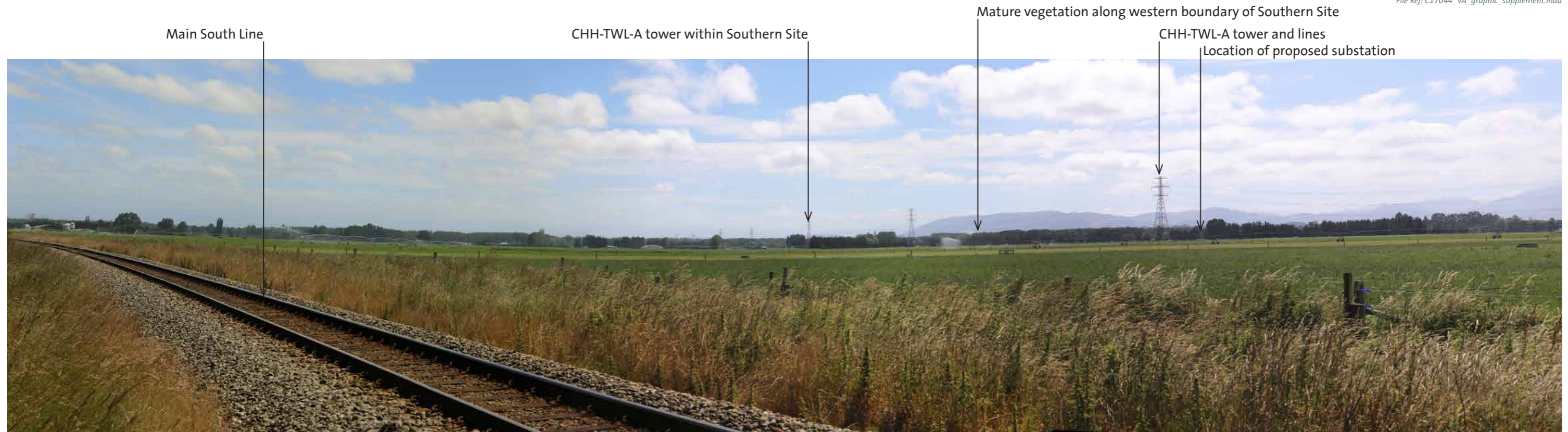
Site Photograph I: Photograph looking west from a location close to the Main South Line towards the Southern Site.
