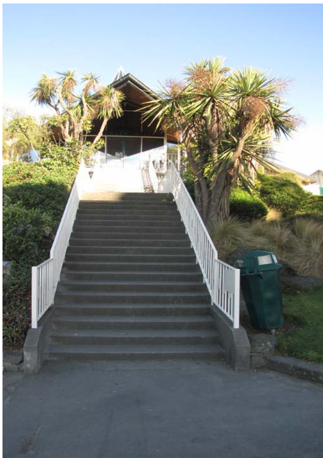
Image above: Public access to the museum via 33 steps from Perth Street.
