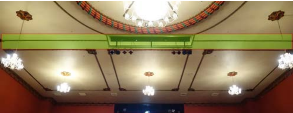
Figure 2: FOH Lighting Bridge with desired extent shaded in green
