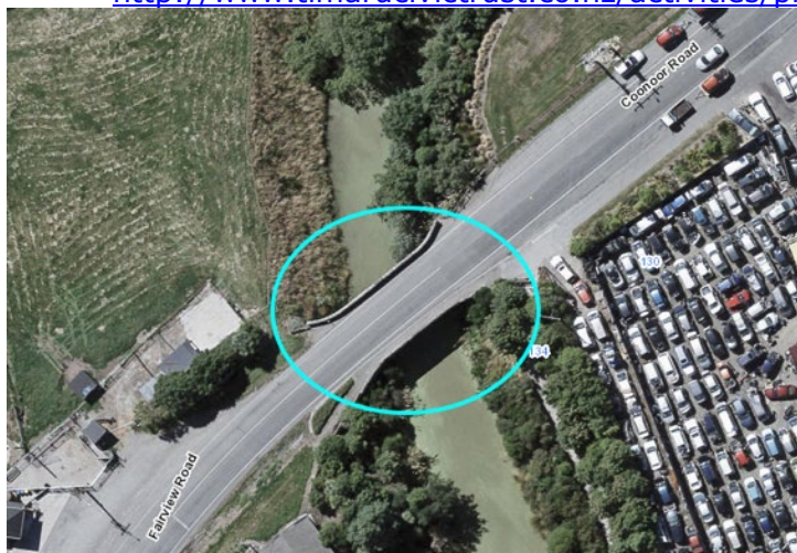
Extent of setting, bridge over Saltwater Creek, Coonoor/Fairview Roads, Watlington, Timaru.
