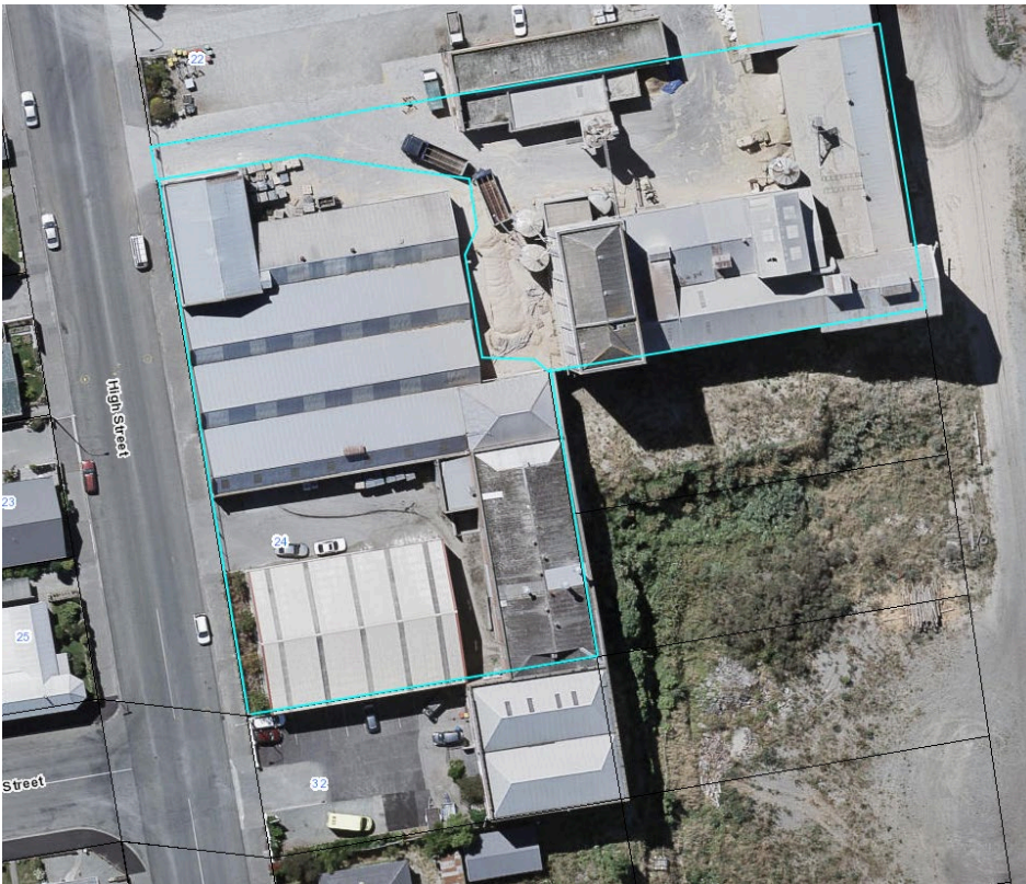
Extent of setting, 24 High Street, Timaru.
