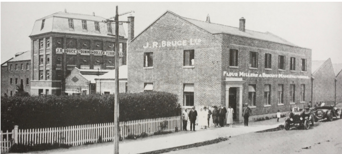
Mid/late-1920s view of JR Bruce's flour mill and biscuit factory. Note mansard roof on flour mill building, this was not reinstated after the 1941 fire. Pan-1481-F, Alexander Turnbull Library, Wellington.
