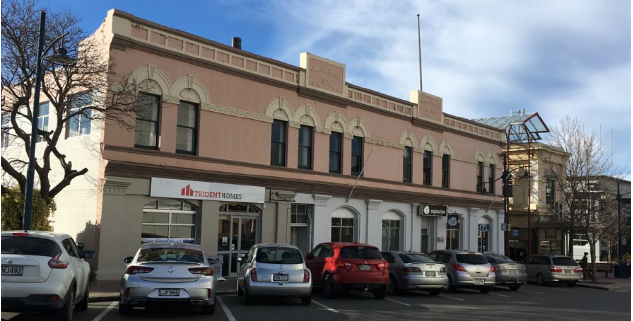
Former Timaru Herald building, 1885-86. Meason & Marchant, architects; Jones & Palliser, contractors. Extended along the Arcade (1906, James Turnbull, architect); extended north along Sophia Street (1928); new press room and paper store built at rear (1954). Dr A McEwan.
