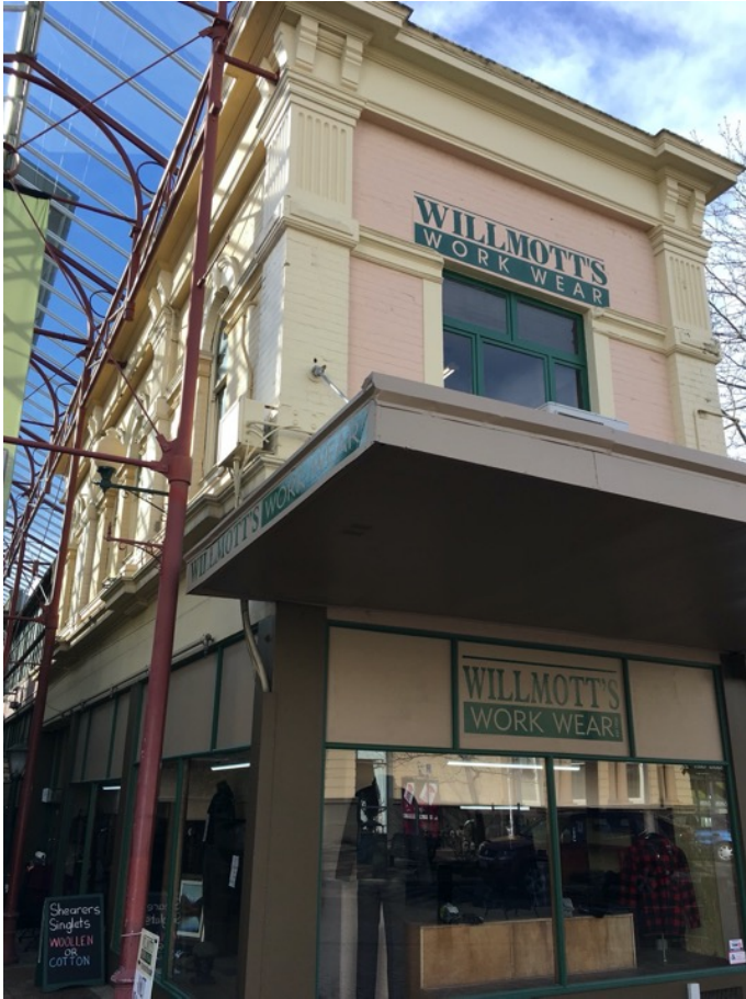
Former United Friendly Societies' (UFS) Dispensary. Maurice Duval, architect. Dr A McEwan.
