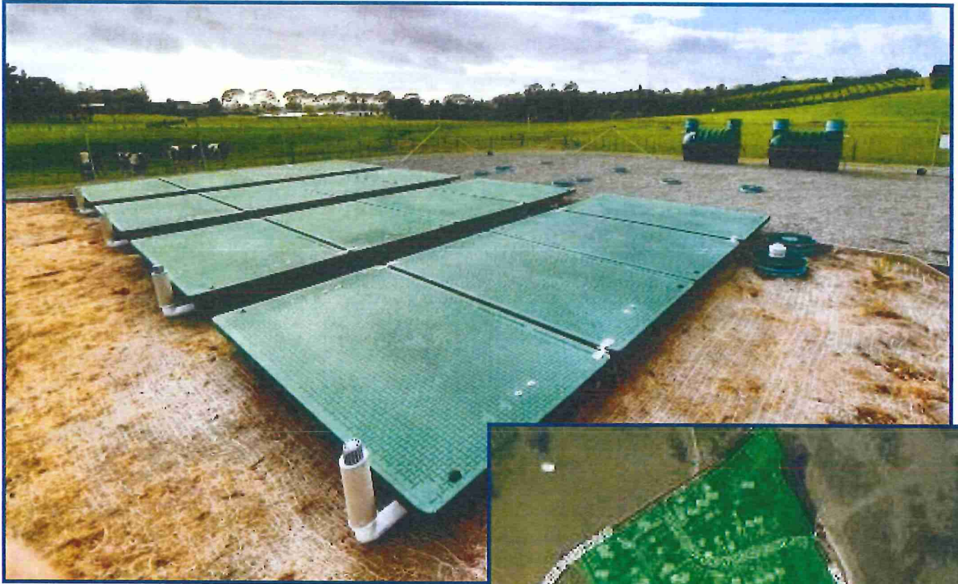
Figure 7-Photo of AdvanTex wastewater treatment plant installed to service the Ongare Point community
