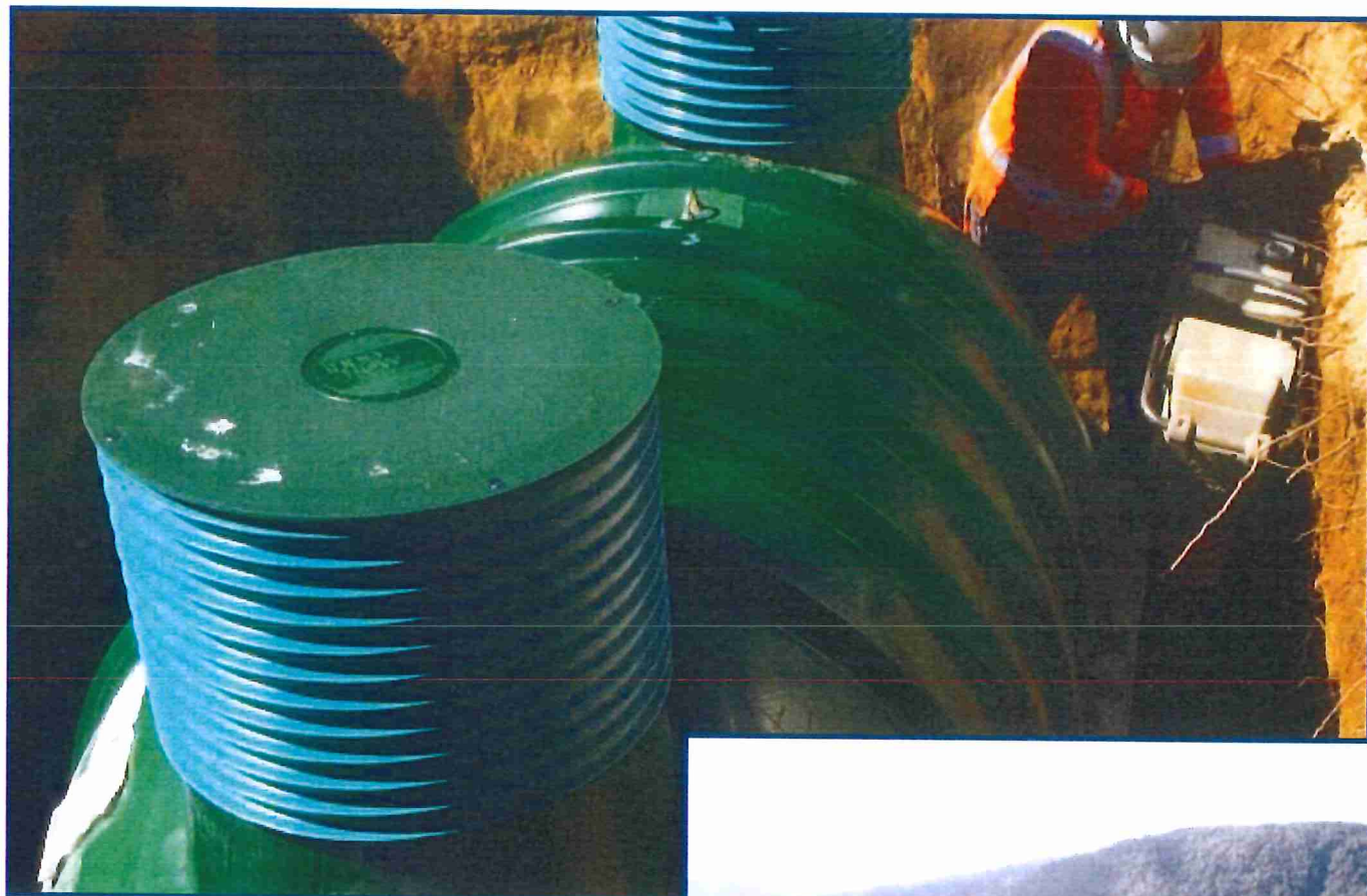
Figure 19-Photo of on-lot tank being installed
