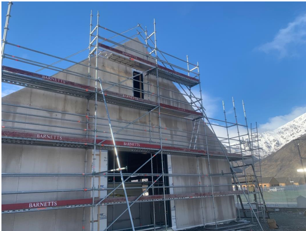
Figure 7 Photograph scaffold with outriggers, credit: Wain Chambers
