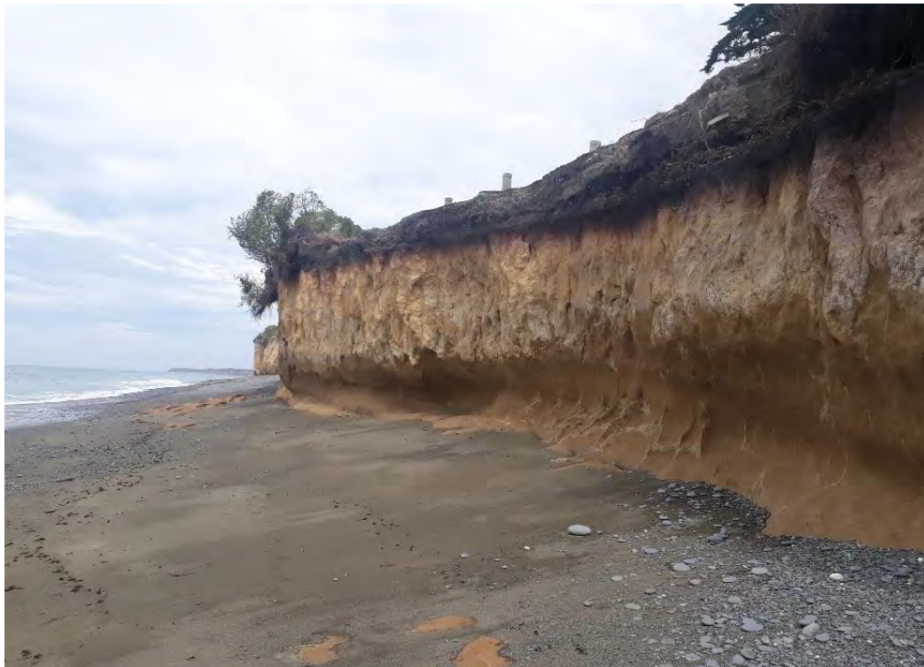
Figure 4: Showing cliff erosion at South Street, Patiti Point, 19 February 2019
