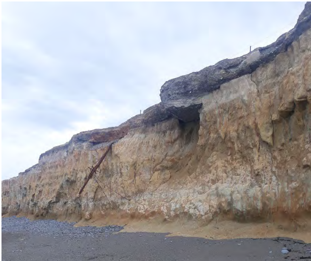
Figure 5: Showing cliff erosion at South Street, Patiti Point, 19 February 2019
