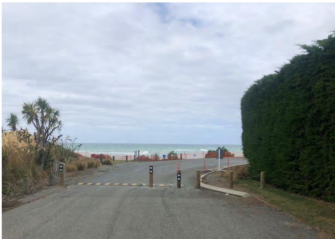
Figure 7: South Street Barrier and Gate, 19 February 2019
