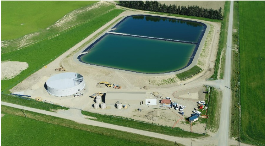
New water treatment plant, water treatment reservoir and raw water reservoir
