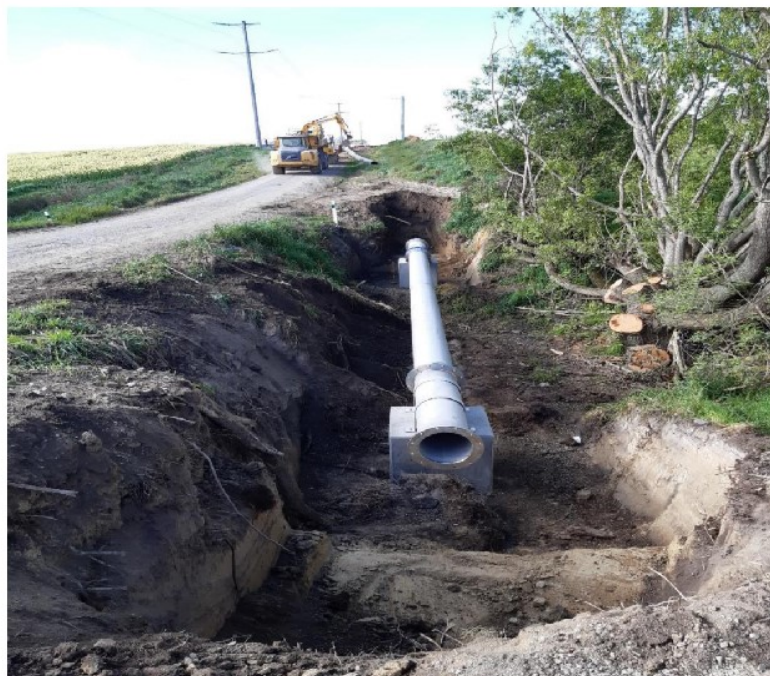
Contract 2470 – Creek crossing installation in George Ward Road
