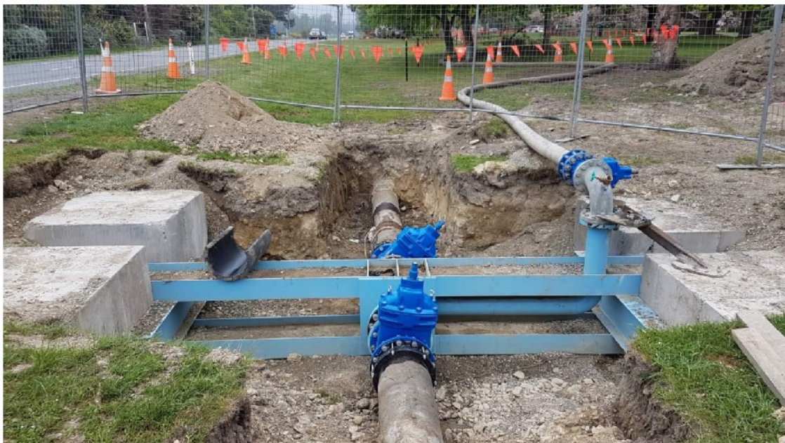
Contract 2338 – Temporary water bypass completed in last lining section in Cave.
