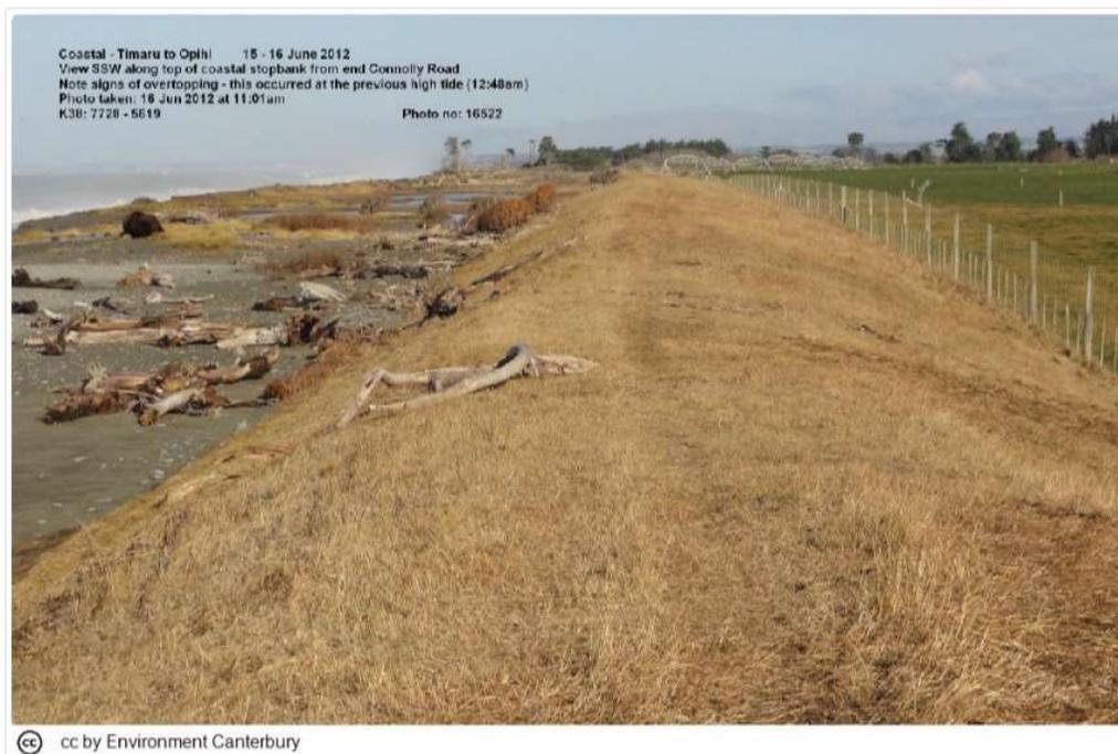
**Figure 2-5: Debris left on stopbank south of Connolly road following June 2012 storm.**Source: ECan.
