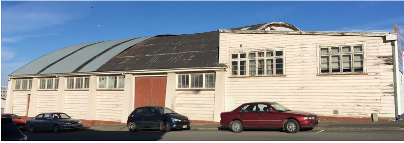
North elevation. Dr A McEwan, 11 July 2018.
