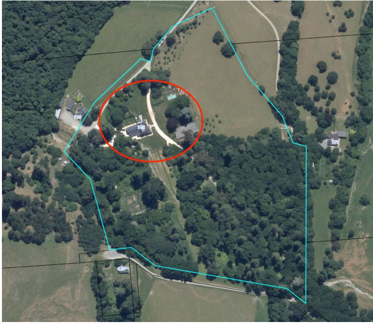
Extent of setting, limited to immediate garden environs, notwithstanding the potential archaeological values across the entire site, 775 Rangitata Gorge Road, Mount Peel, Peel Forest.
