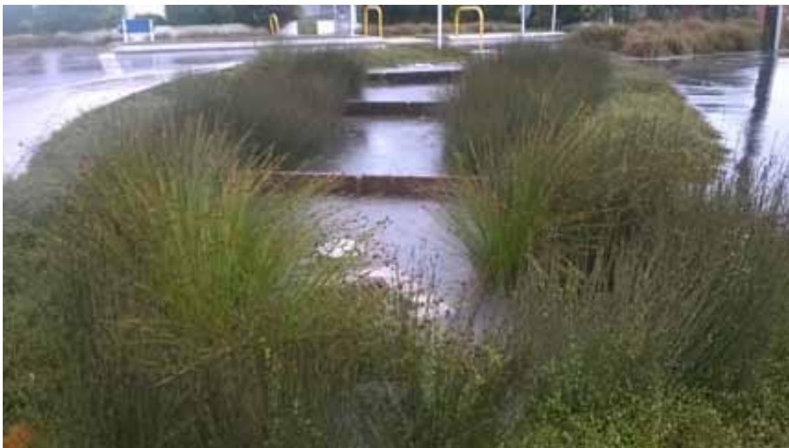
Morgan's Road Rain Garden – Stormwater management techniques
