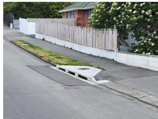
Fig. 79: A recent sump renewal in urban Timaru, to address flooding issues in this flooding depression area. This asset will rely on the capacity of stormwater mains at this location which were not renewed.
