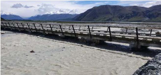
Fig 91: Forest Creek Bridge – high river flows have reduced the extent of Forest Creek Bridge, and caused significant damage to one of its piers during the 2021 flood event.
