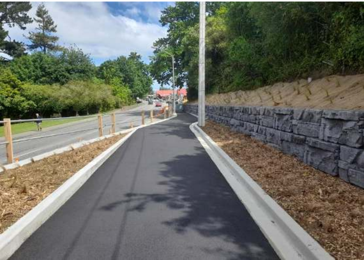
Fig 90: Coulter Place, Geraldine – a new retaining wall has been installed in 2023. This was an important resilience upgrade for State Highway 79, but funded by Council due to proximity to the footpath.
