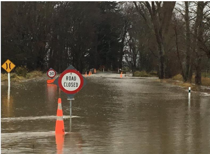
Fig. 92: Flooding at Langridge Road bridge – we have received resilience upgrade requests for this location. The existing structure is not near the end of life, if project was to be brought forward it would require full Council funding including a full assessment of flow paths.
