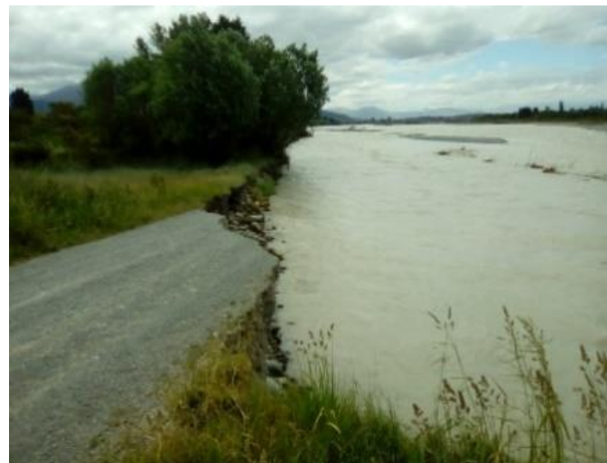
Fig. 67: Ferry Road, Arundel – During the December 2019 flood event that closed all connecting bridges across the Rangitata River and temporarily severed the South Island in two, the Rangitata River flow diverted onto road reserve and forced the abandonment of a large section of Ferry Road. In the time since this event, the river has not diverted back to previous channels and this section of road remains closed.
