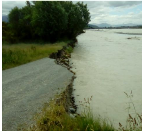
Fig. 19: Ferry Road – Arundel – During the 2019 flood event that closed all connecting bridges across the Rangitata River and temporarily severed the south island in two, the Rangitata River flow diverted onto road reserve and forced the abandonment of a large section of Ferry Road.
