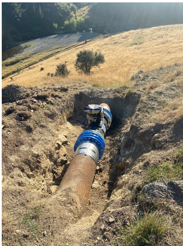
Contract 2469– Pareora Pipeline Renewal Section 2
