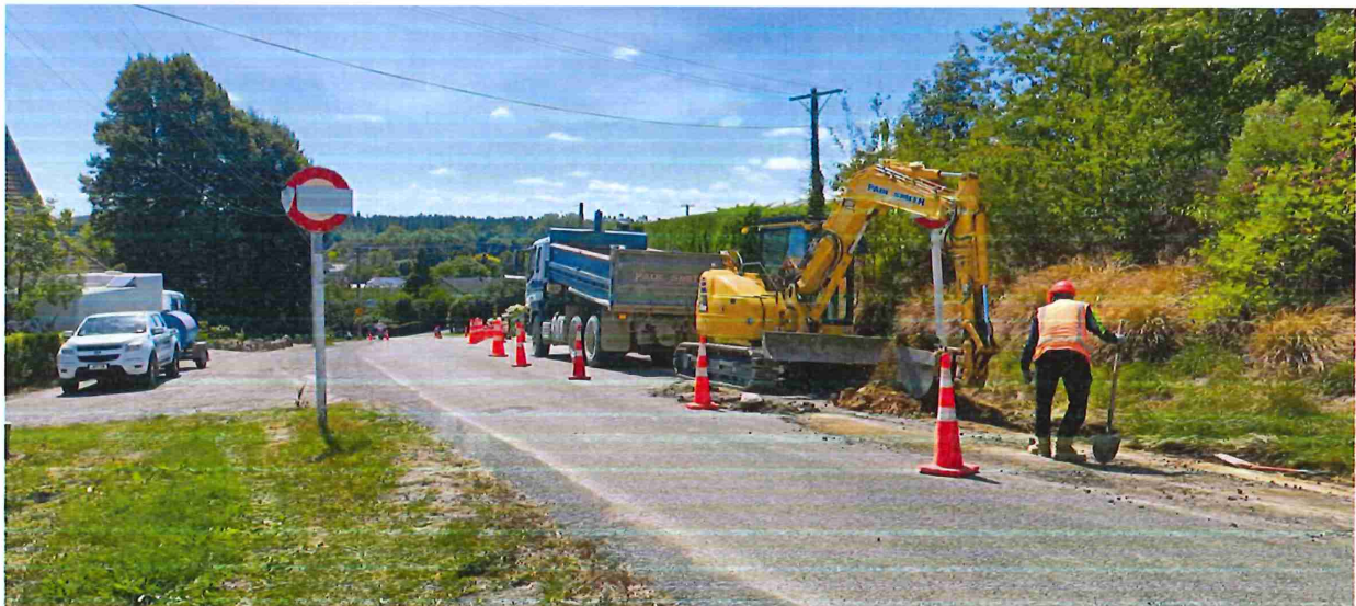
Construction in Progress – Manse Road, February 2024
