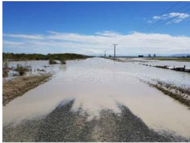
3. Old Main South Road looking South
