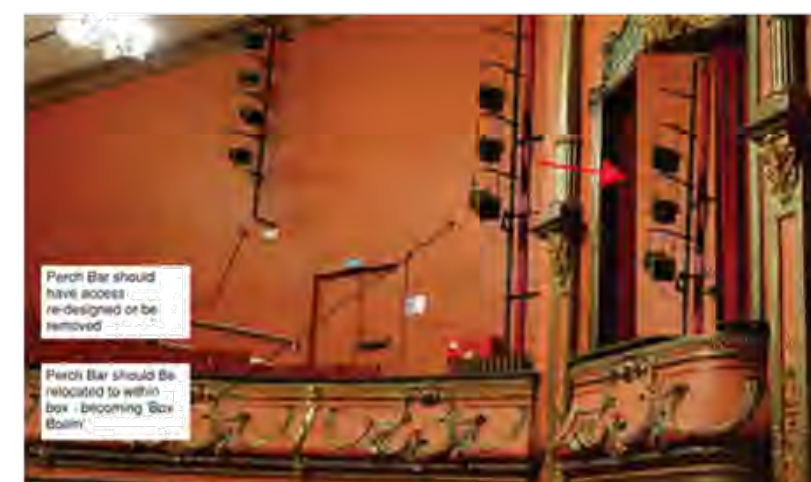
Figure 3: Perch bar redesign requirements
