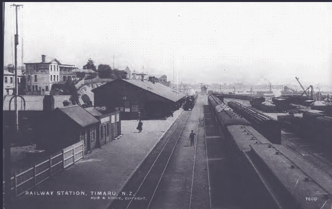
Timaru Railway Station.
