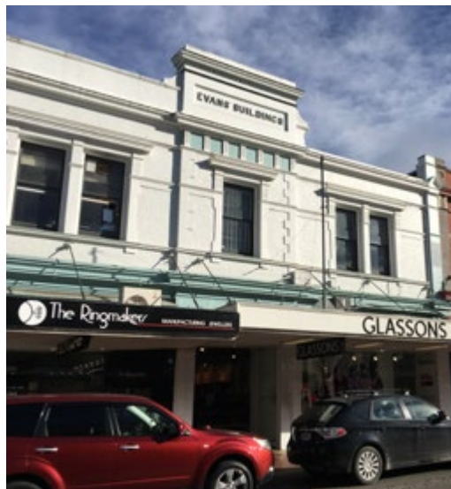
Figure 40: Evans' Buildings [detail], 266-272 Stafford Street, 1904. Dr A McEwan.
