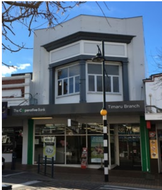
Figure 48: Commercial building, 295 Stafford Street, 1928. Dr A McEwan.
