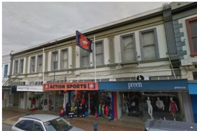
Figure 33: Durand's Buildings, 202-210 Stafford Street, 1869 + c.1875.
