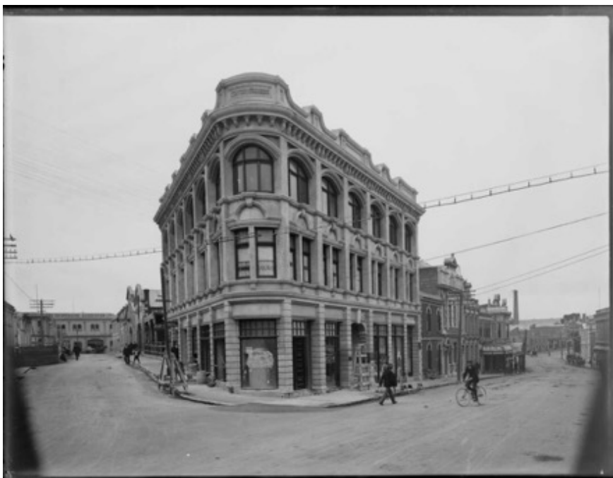
Figure 10: Stafford Chambers nearing completion, c.1908. 1/1-008714-G, Alexander Turnbull Library, Wellington.
