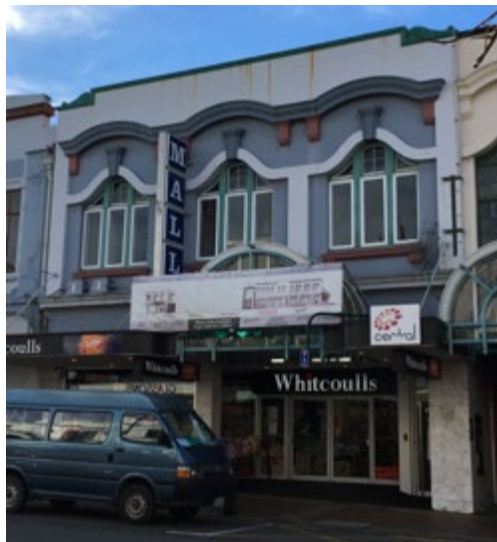
Figure 41: Commercial building, 269-71 Stafford Street, 1917. Dr A McEwan.
