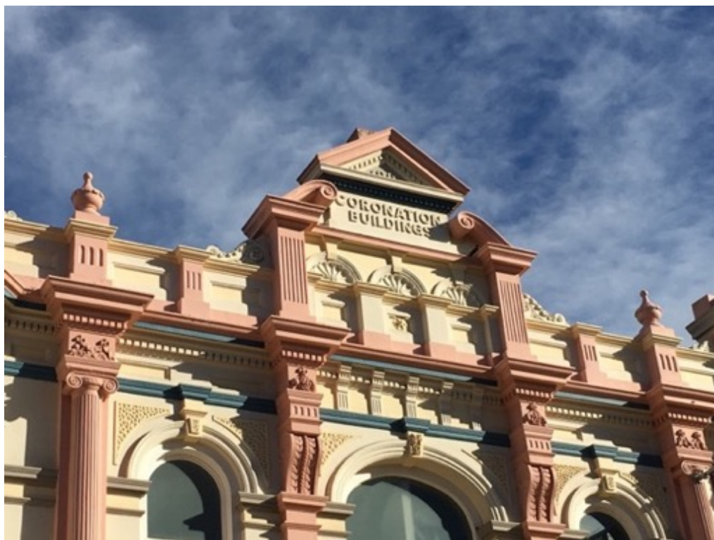
Figure 2: Detail of Coronation Buildings, Stafford Street, Timaru. Dr A McEwan.
