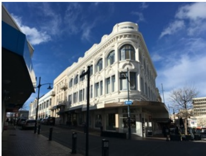
Figure 12: Stafford Chambers, 199-209 Stafford Street / 18-22 Beswick Street, 1908; Thomas Coulthard Mullions, architect; HN Hollow, builder. Dr A McEwan.
