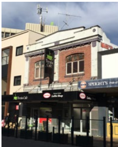
Figure 21: former Mays Bakers, 160-162 Stafford Street, 1928. JG Broadhead, contractor. Dr A McEwan.
