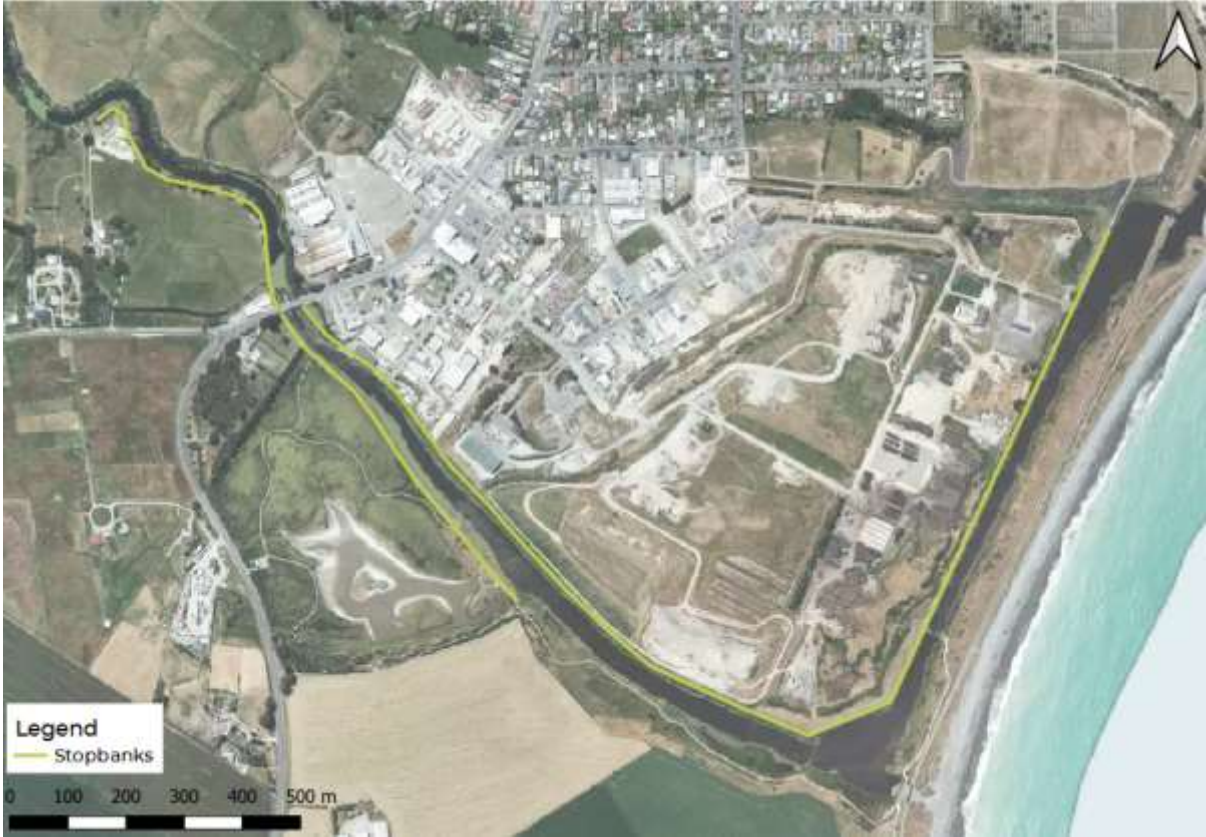
Figure 5-13 Stopbanks along Saltwater Creek
