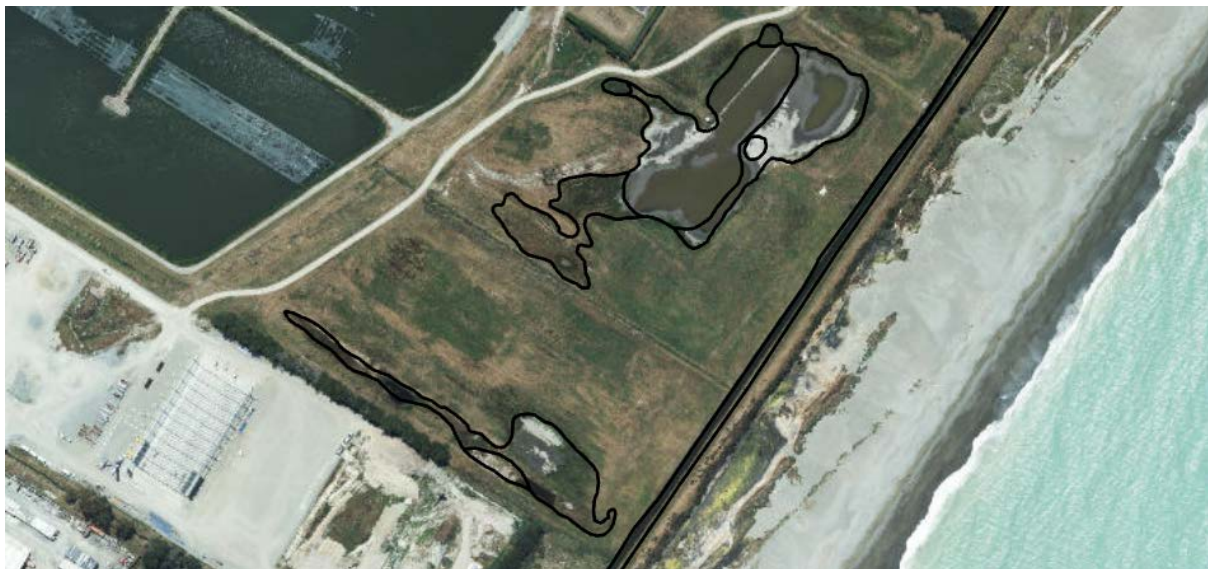
Figure 4 The existing extent of the 'pit-derived wetlands' south of Aorangi Road. These wetland areas, considered 'natural inland wetlands', were induced following earthworks associated with the adjacent water treatment ponds.
