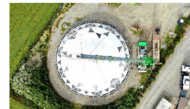
Temuka Treated Water Reservoir – Top view
