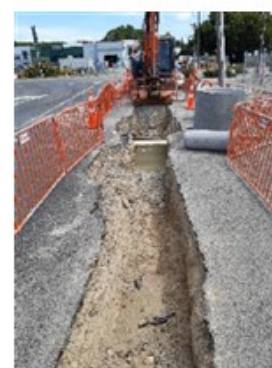
Fraser Street Stormwater Upgrade - Temuka
