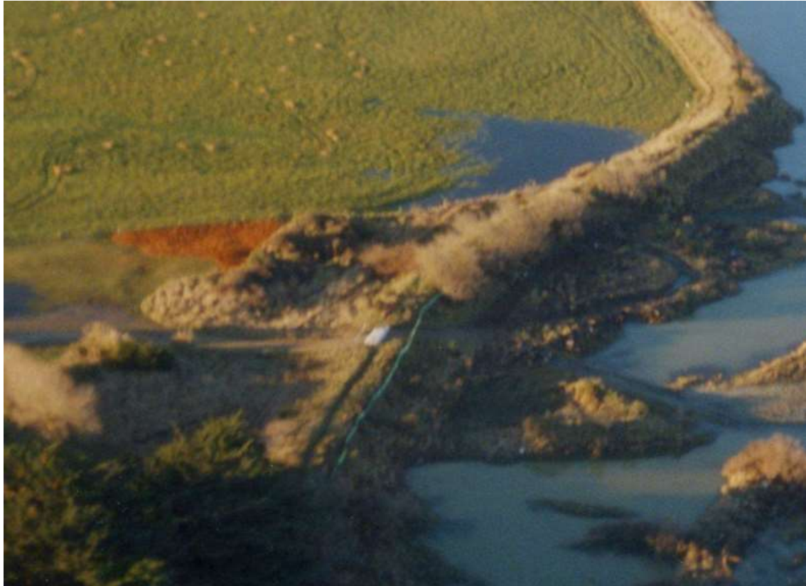
Figure 2-3: Sandbags (white) placed on the Milford Hut stopbank during the 2001 Storm. Source: ECan.
