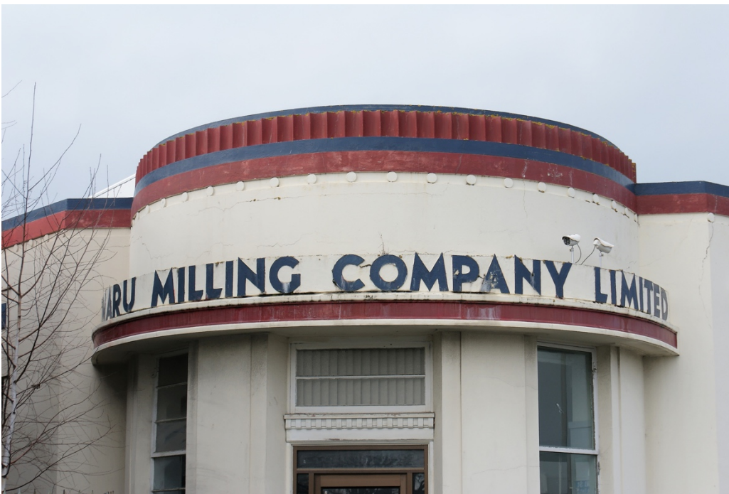
Building detail. Dr J Wilson, 12 September 2018.
