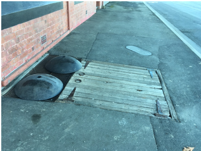
Cellar access on Main Road footpath. Dr A McEwan, 12 July 2018.
