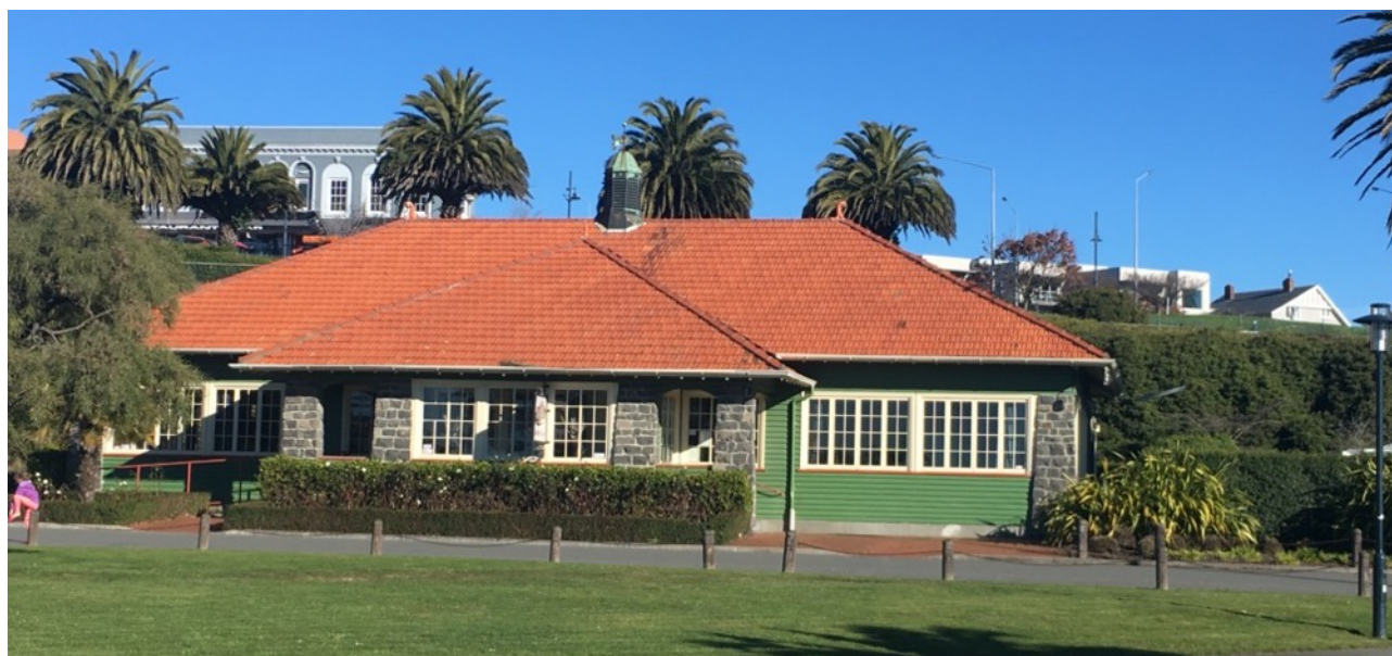
Figure 16: Tearooms ([1905/1907/1913/1920] 1931; FW Marchant (1905), Walter Panton & Son (1913 & 1931), Harold Broadhead (1920), and Turnbull and Rule (1931), architects; Messrs Stoddart & Mitchell, builders (1931).
