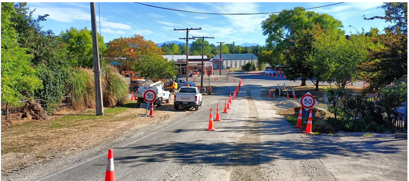
Construction in Progress – Manse Road, March 2024
