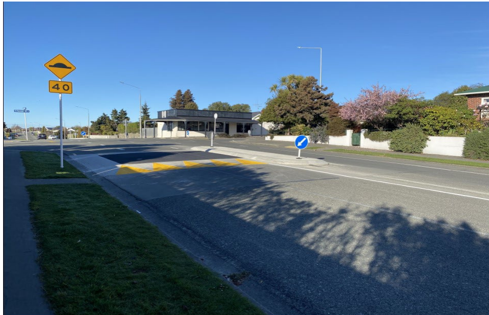
Woodlands Road – Hassall Street – Raised Safety Platform and Traffic Island (Southbound Lane)
