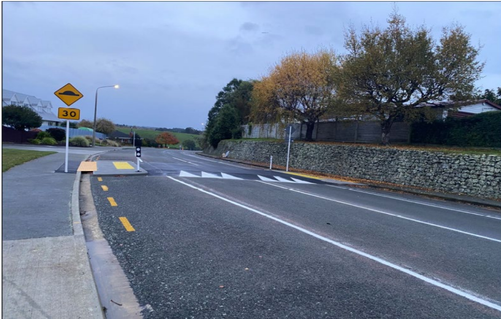
Quarry Road, Timaru – Midblock Raised Pedestrian Crossing
