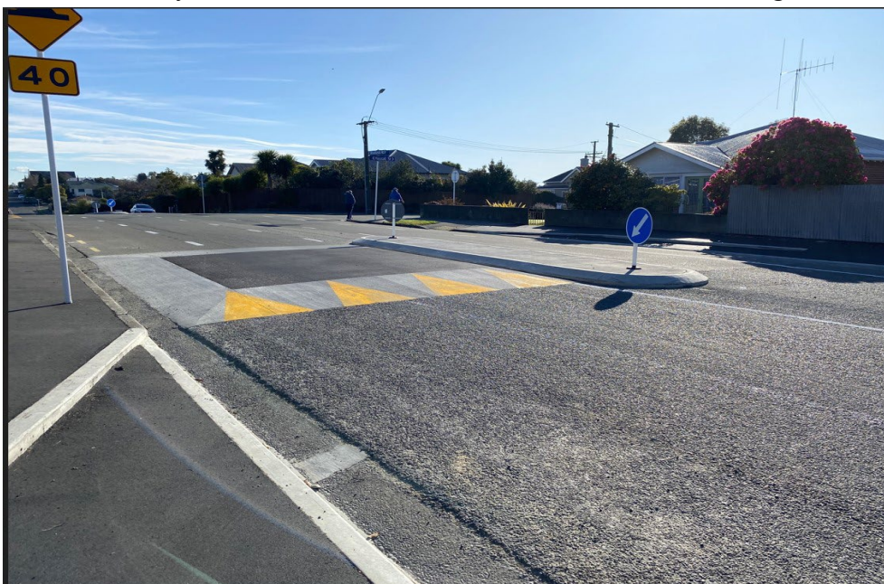
Woodlands Road – Hassall Street – Raised Safety Platform and Traffic Island (Northbound Lane)
