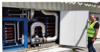
Action Friction shows part of the brewery refrigeration system, using ammonia as refrigerant in an outdoor-cooled unit. The oil is transferred by heat exchanger to less-hazardous glycol for piped circulation through the plant.
