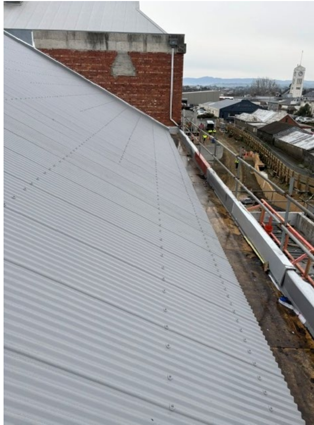
Auditorium roof replacement
