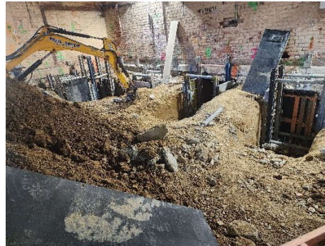
20260609_ASVR12_07 - Stage house excavation and underpinning
