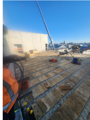
20260630_100925 - Museum first floor structure / rib preparation
