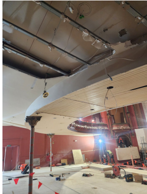
20260626_112529 - Auditorium floor / ceiling works
