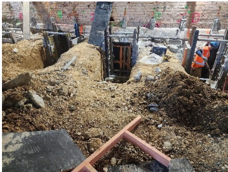
20260609_ASVR12_08 - Stage house foundation preparation
