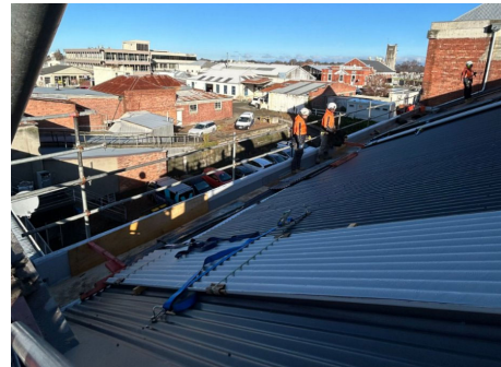
20260616_ASVR13_12 - Auditorium roof replacement works
