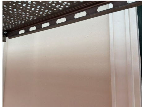
20260619_ASVR14_14 - Facade cladding and finish check
