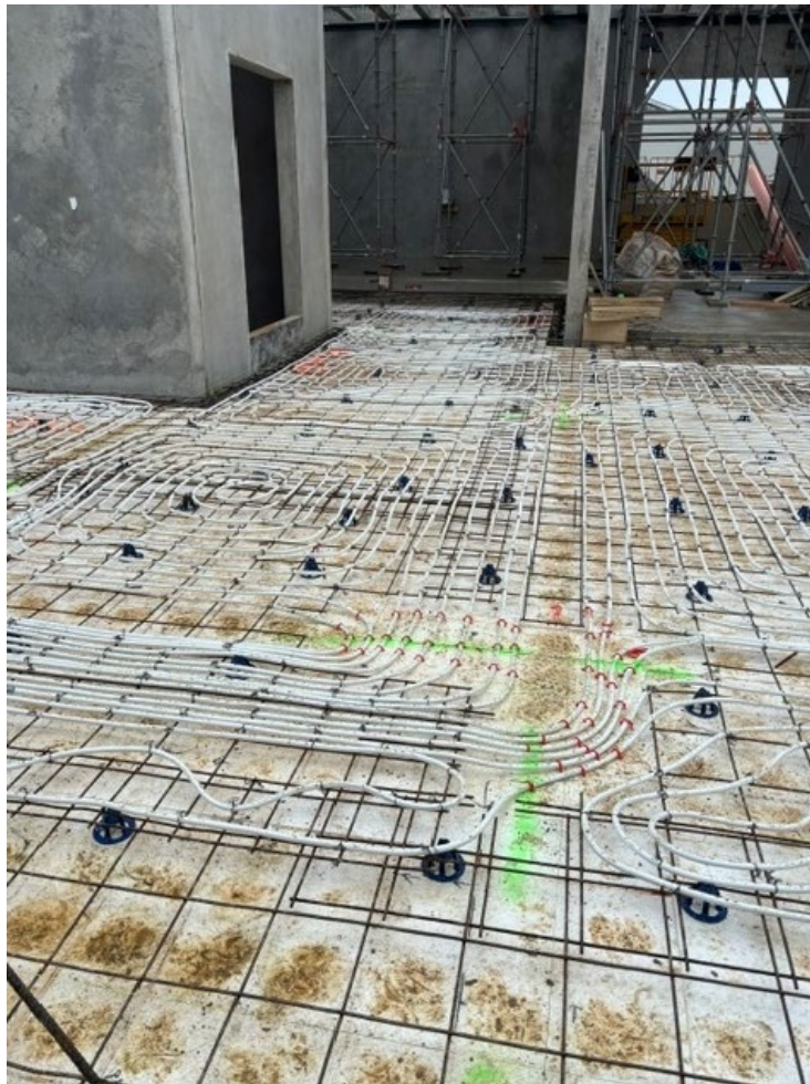
Underfloor heating installation to museum lobby / entry
