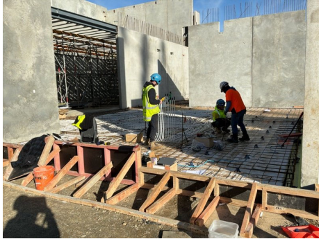
20260623_ASVR15_16 - Museum first floor structure / Stahlton
