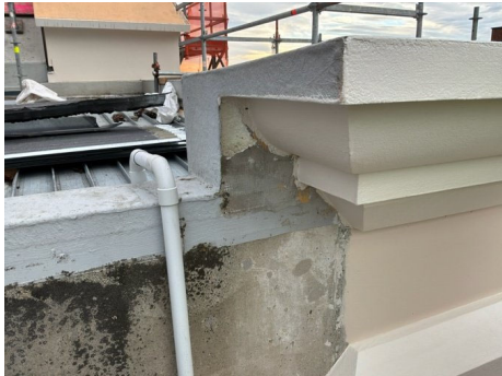
20260619_ASVR14_13 - Parapet and facade making good
