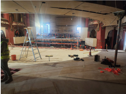
20260630_103608 - Auditorium floor structure works
