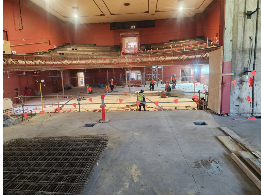
20260630_111608 - Auditorium floor works
