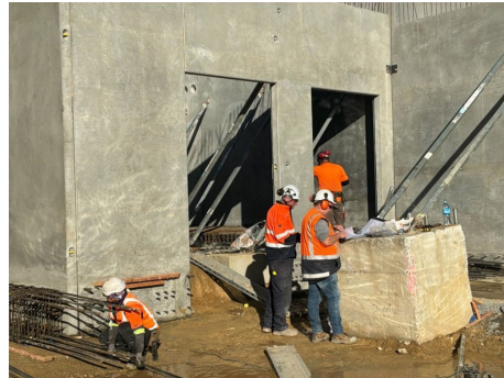
20260623_ASVR15_11 - BOH precast installation
