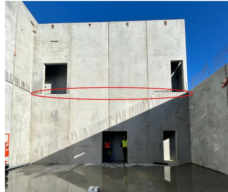
20260616_ASVR13_04 - Museum precast panel installation
