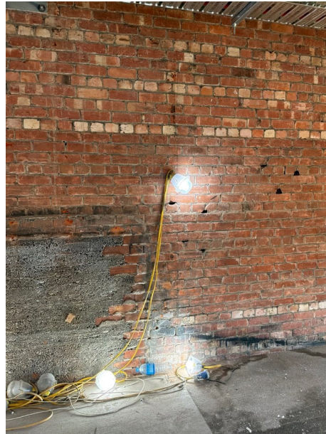
20260630_ASVR16_05 - Existing brick opening / structural review
