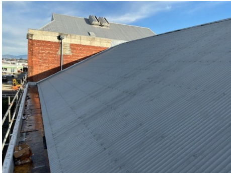
20260623_ASVR15_10 - New corrugate roofing
