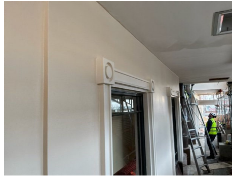
20260619_ASVR14_10 - Stafford Street facade preparation
