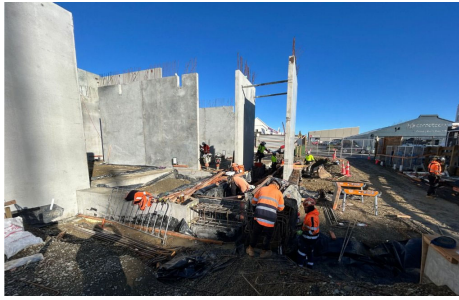
20260616_ASVR13_02 - BOH precast panel and ground works
