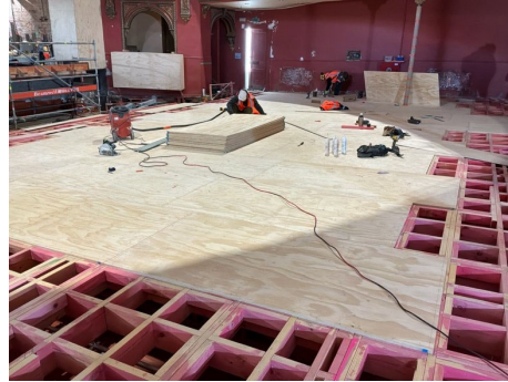
20260623_ASVR15_06 - Auditorium plywood installation
