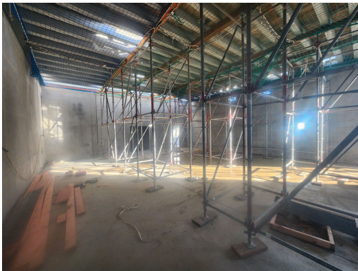
20260630_101041 - Museum scaffolding / internal works
