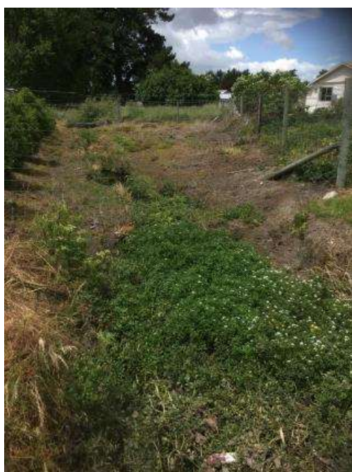
D12 Serpentine Creek Channel Downstream Kennedy Street
