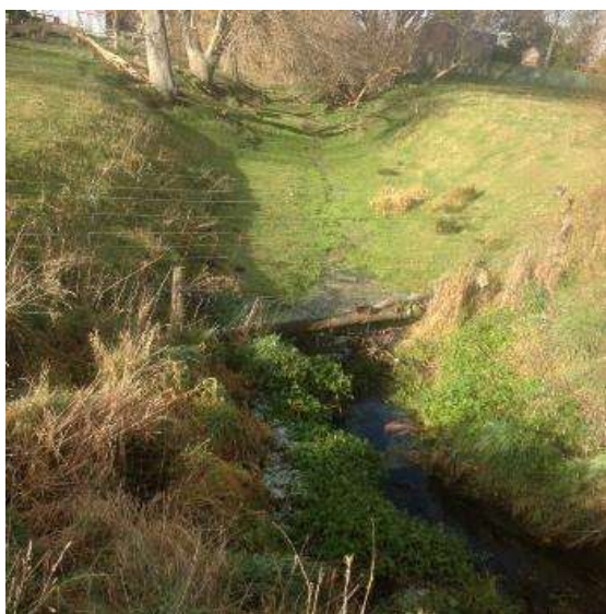
D14 Serpentine Creek Channel Downstream Winchester- Geraldine Road
