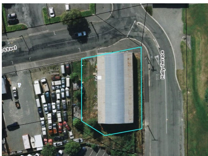
Extent of setting, corner of Commerce Street and Hally Terrace, Temuka.
