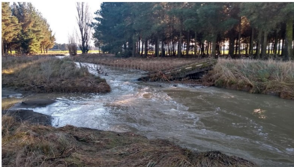
Seaward Road Bridge
