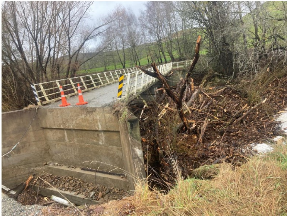
Hall Road Bridge
