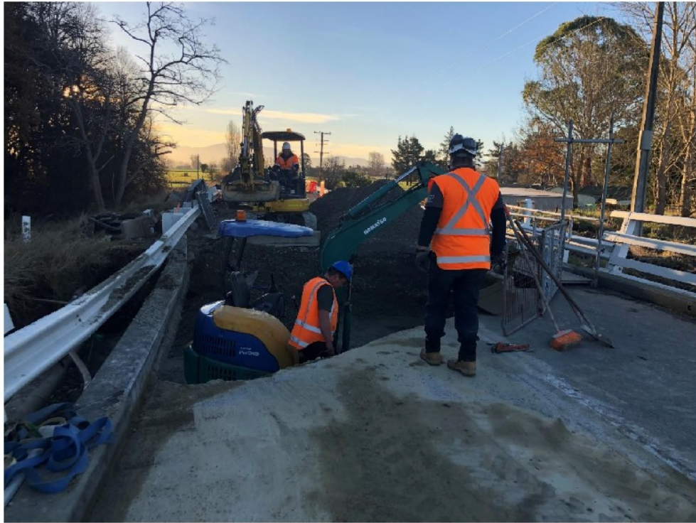
Repairing the Waihi Bridge
