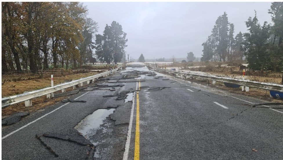
Coopers Creek Bridge on R72 Geraldine Arundel Rd
